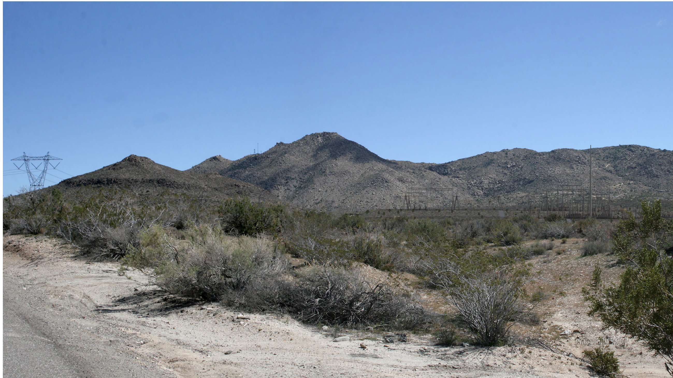
Visual simulation from Old Highway 80 - ECO Substation with landscaping at 5 years of maturity
