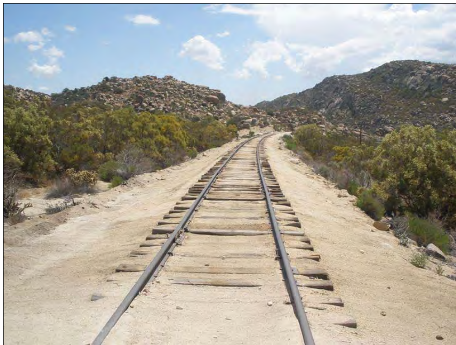
FIGURE 5-46. SAN DIEGO ARIZONA RAILROAD SEGMENT
