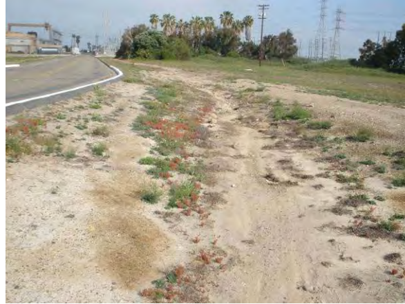
Roadside drainage depicting higher flow evidence within a swale lacking defined channel banks.
