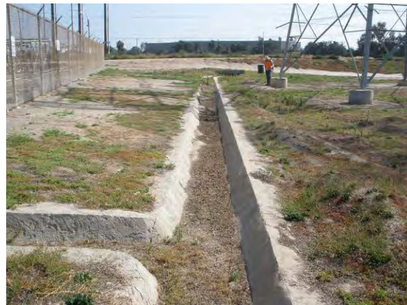
Concrete-lined ditches draining stormwater from substation yard.
