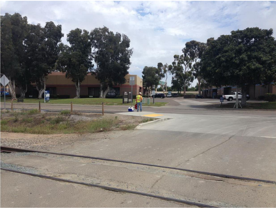
Photo 6: Traffic Control flaggers were stationed at the entrance of the Bay Boulevard Substation site during heavy oversized load deliveries in accordance with the Traffic Management Plan (APM-TRA-01).
