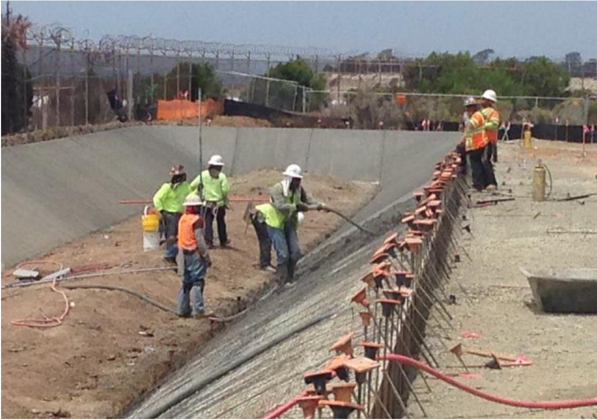
Photo 3: Pouring concrete along the slope of the bioswale (western edge, above).
