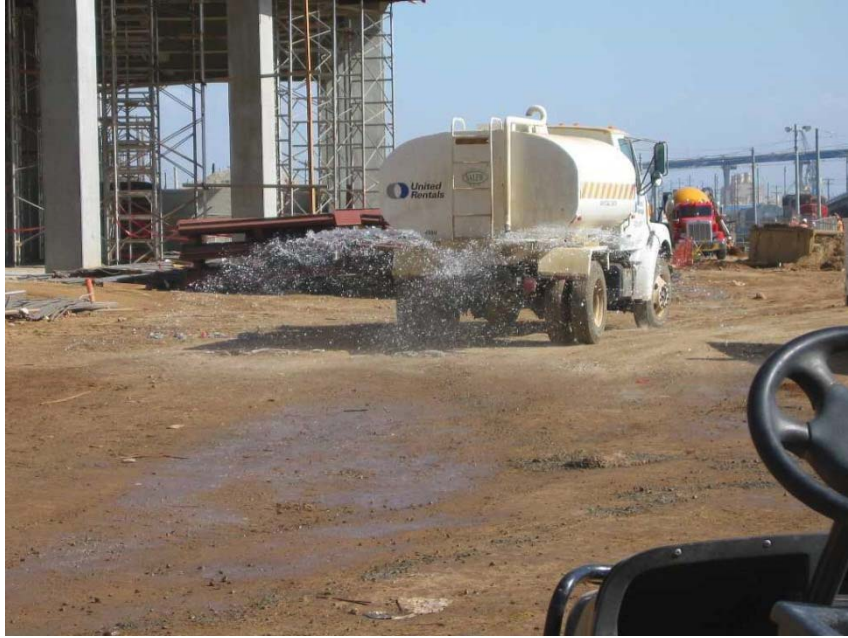
Water being applied for dust control.
