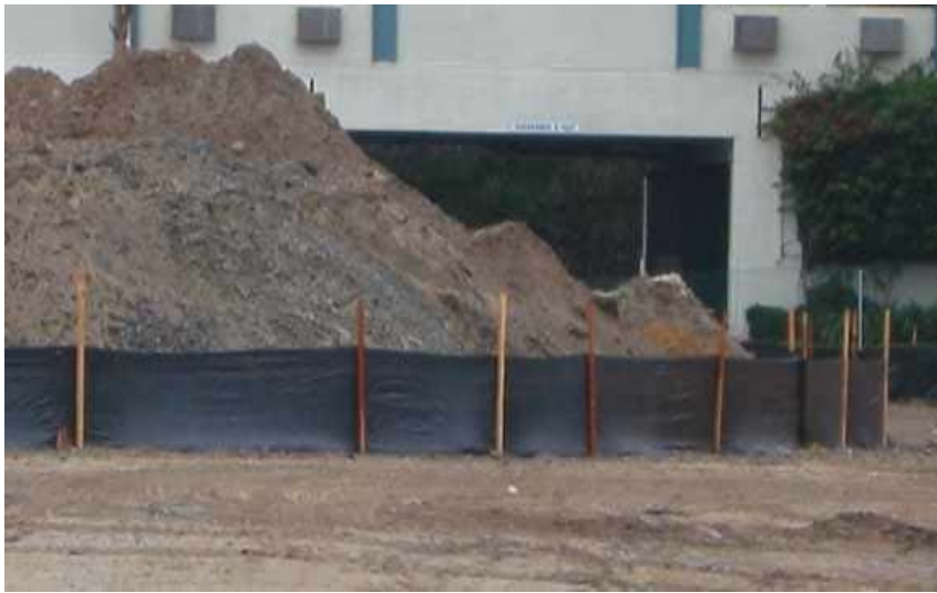
Silt fence used for stockpile perimeter control.
