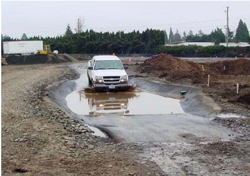
Drive through wheel wash before exiting a site.
