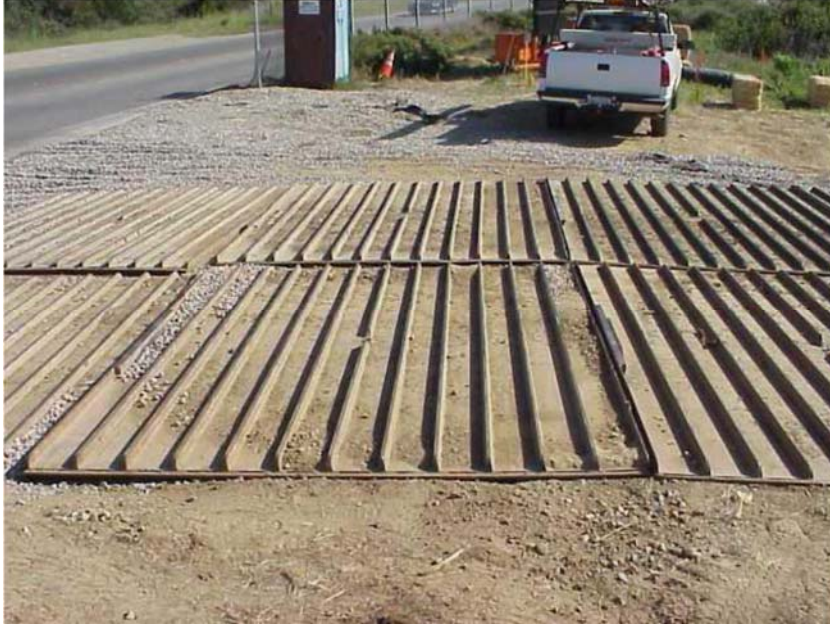
Manufactured metal plates knock dirt off vehicle tires before exiting a site.
