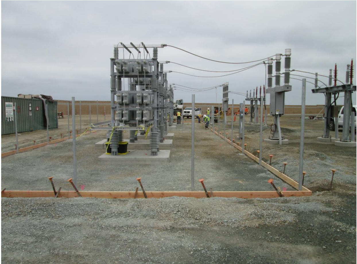
Photo 2: Crews were observed preparing to pour concrete within the 230kV yard.
