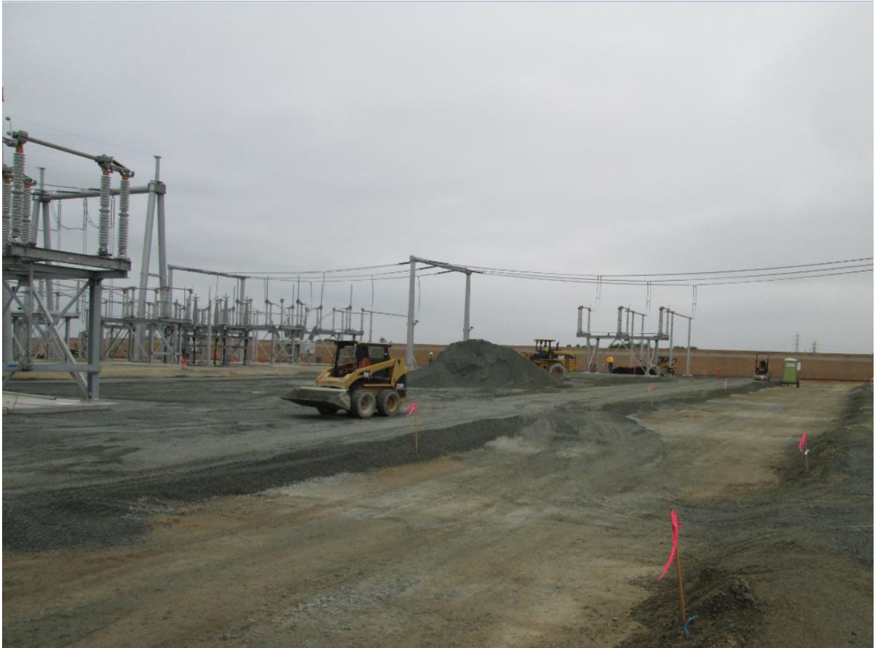
Photo 1: Crews were observed placing Class II base within the Bay Boulevard Substation.
