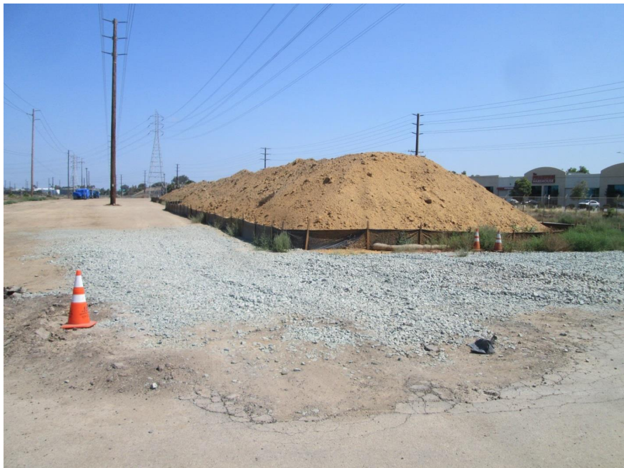
Photo 3: Erosion and sediment control BMPs, such as the use of silt fencing around the pictured stockpile, were observed being implemented on-site in accordance with the project SWPPP (MM-HYDRO-01).
