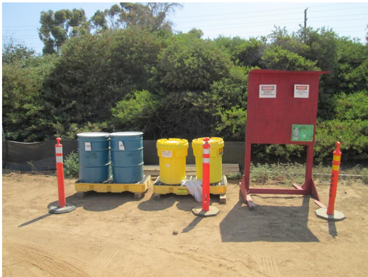
Photo 4: In accordance with HSMERP (APM-HAZ-01), the hazardous materials staging area included the use of labeling, containment units, and the staging of spill kits.
