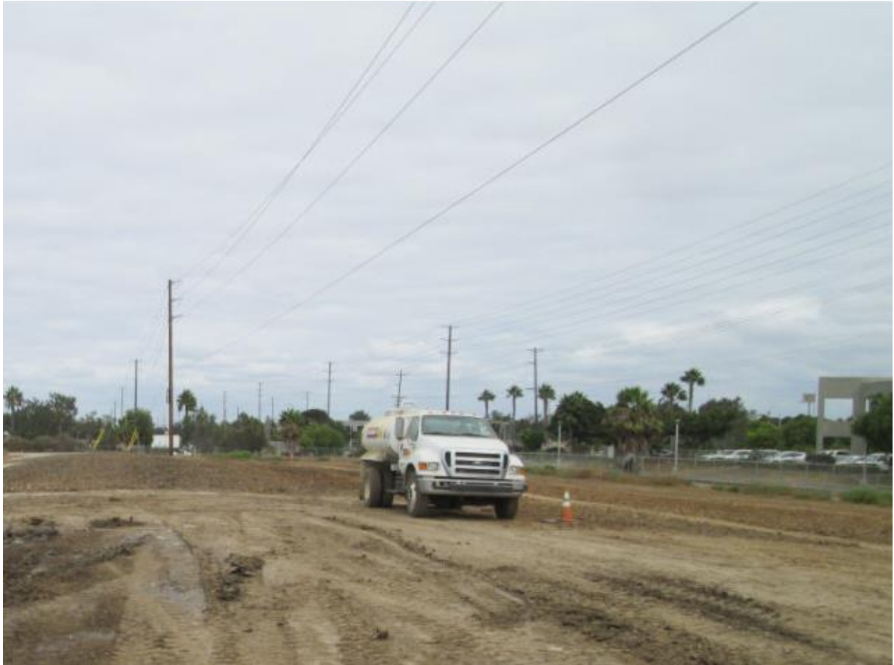
Photo 2: Water trucks were observed applying water to work areas to minimize fugitive dust in accordance with MM-BIO-5.
