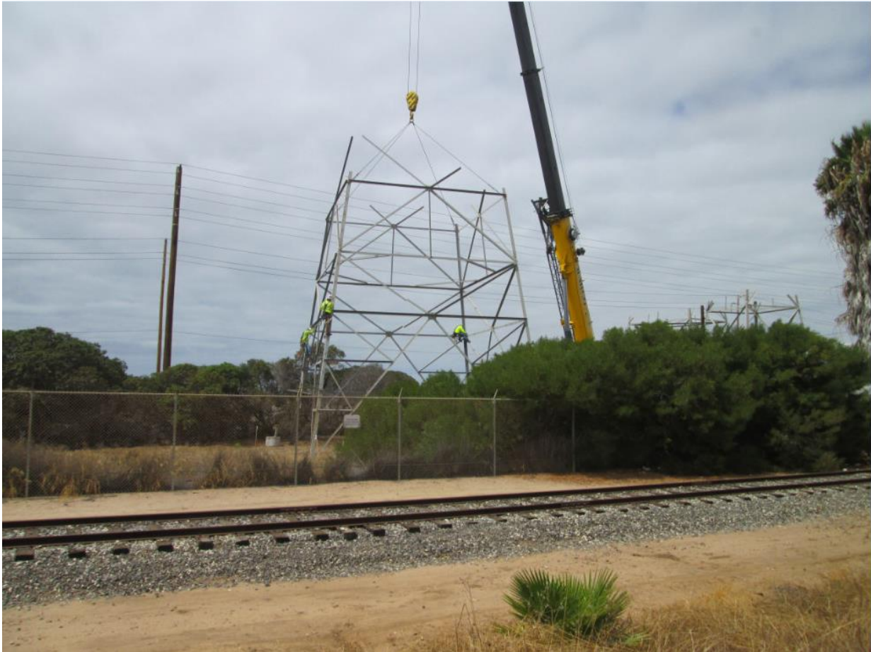
Photo 1: Crews were observed disassembling a lattice tower along the transmission ROW.
