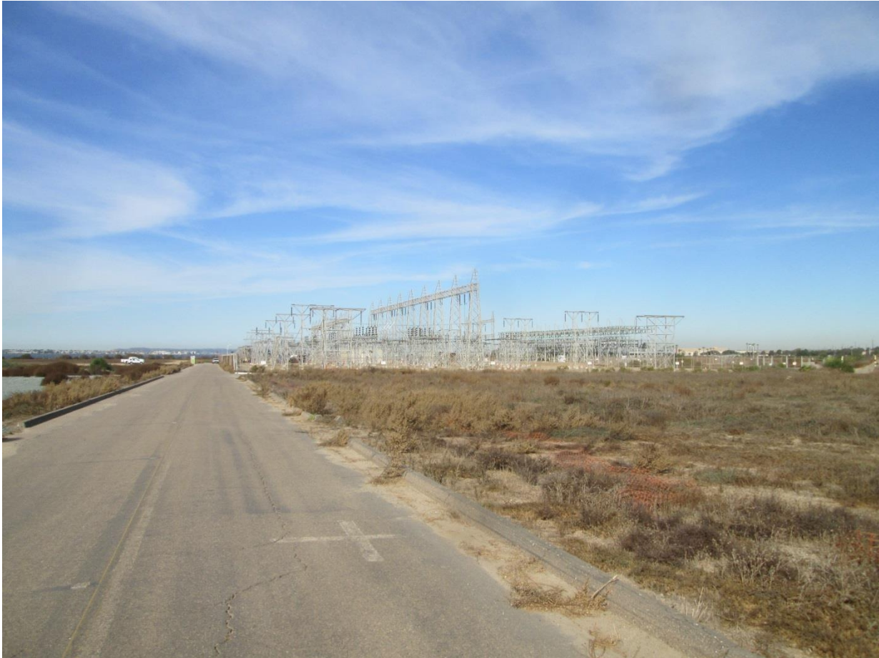
Photo 1: South Bay Substation demolition site in Chula Vista, California on December 5, 2017.
