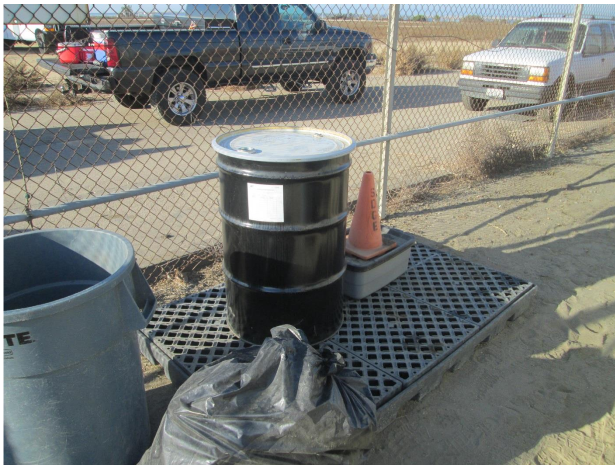
Photo 3: Hazardous materials were staged over secondary containment pallets in accordance with the Hazardous Substance Management and Emergency Response Plan (APM-HAZ-01).
