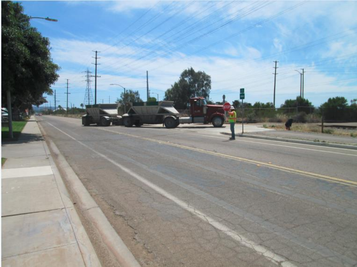
Photo 3: During import of fill material, a traffic-control flag person was utilized to direct traffic along Bay Boulevard and the parallel bike path in accordance with the project Traffic Management Plan (MM TRA-01).
