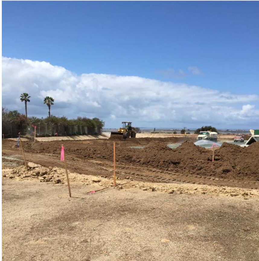
Photo 1: Archaeological monitors observing excavation and re-compaction activities in accordance with MM CUL-01. Water trucks were used to prevent fugitive dust in accordance with APM AIR-01.
