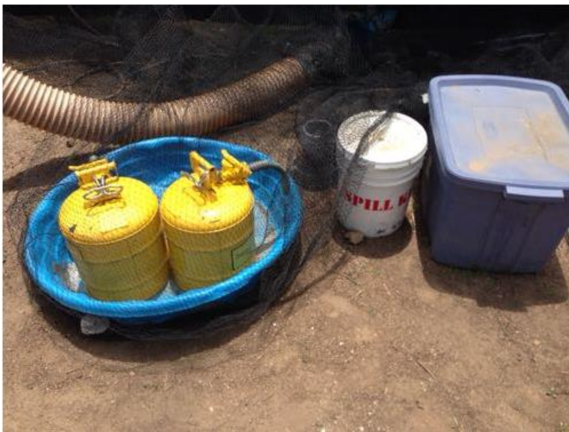
Photo 4: Spill prevention measures included secondary containment bins under equipment, fuel, etc. in accordance with APM-HAZ-01. Spill kits were observed staged throughout the site in accordance with this measure.
