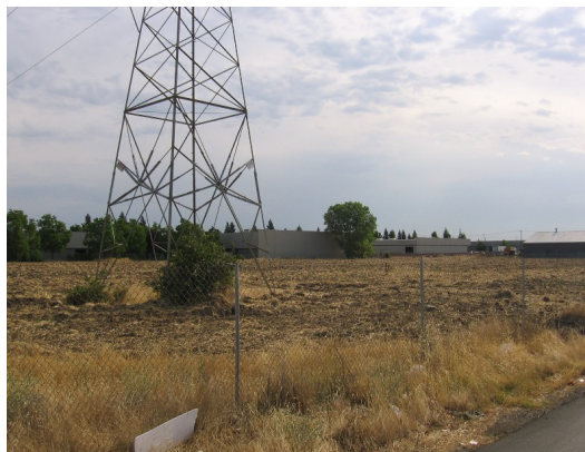
Northeasterly view of wellhead site
