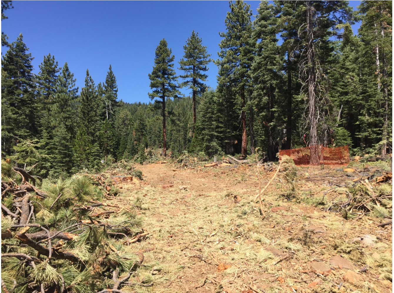
Photo 2: Tree removal work along right-of-way, including nest tree flagging and fencing.
