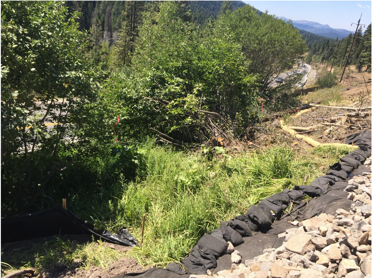
Photo 1: Dry rock ford with erosion control best management practices (BMPs) installed at project access road crossing of Drainage 1208, between Poles 291148 and 291149.
