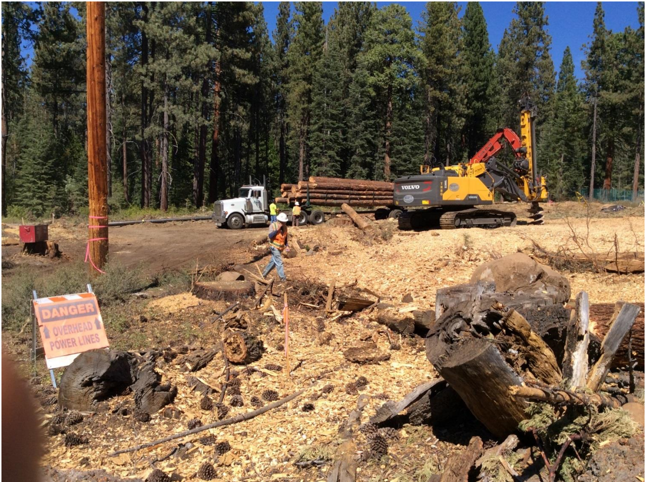
Photo 5: Final log loading for timber operations, at the Kings Beach Substation.
