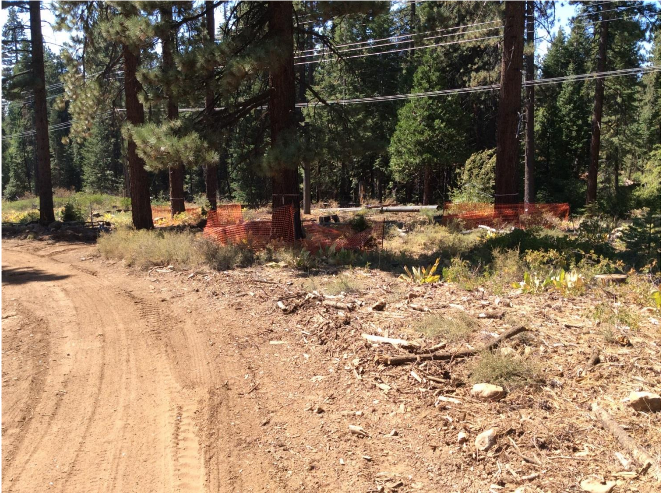
Photo 4: Fencing for retained tree protection, near Pole 291236.
