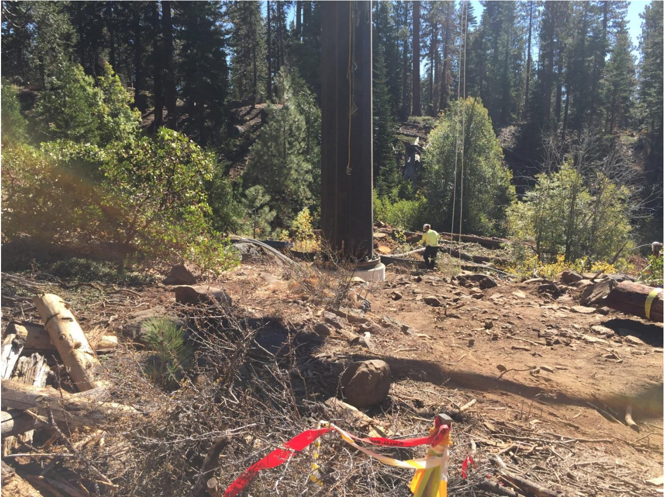
Photo 6: Stringing at Pole 291226, across Griff Creek.
