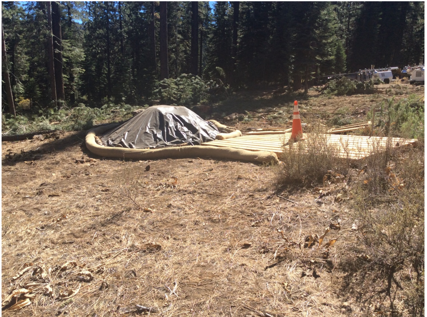
Photo 2: Topsoil stockpiled and covered near Pole #291261, in accordance with APM-BIO-23.
