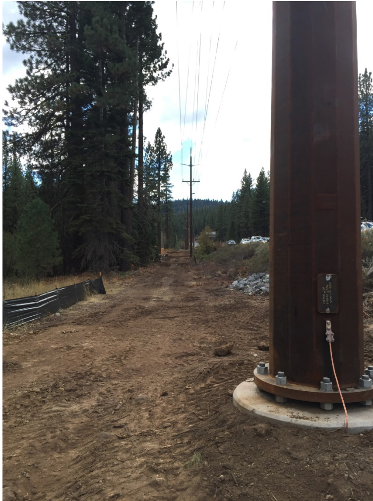
Photo 3: Pole #291105 installed and native topsoil replaced (APM-BIO-23).
