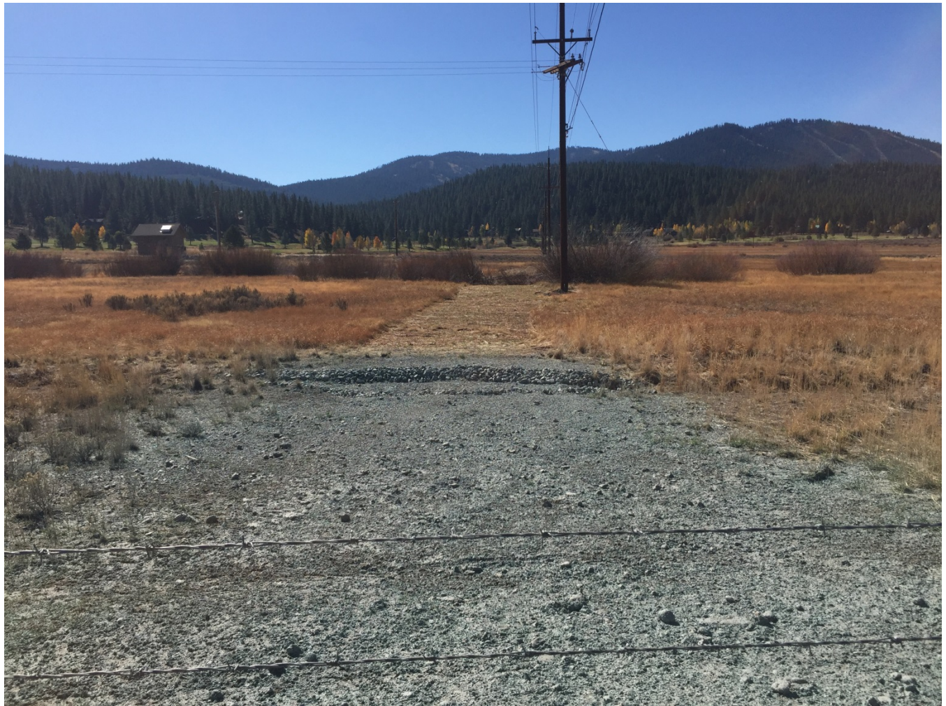
Photo 6: Right-of-way in Martis Valley between Poles #291067 and #291068 following removal of timber matting, timber bridges, equipment, and materials. Disturbed areas hydro-seeded and areas where timber matting had been used hand-seeded. The ROW has been fenced to prevent unauthorized access.
