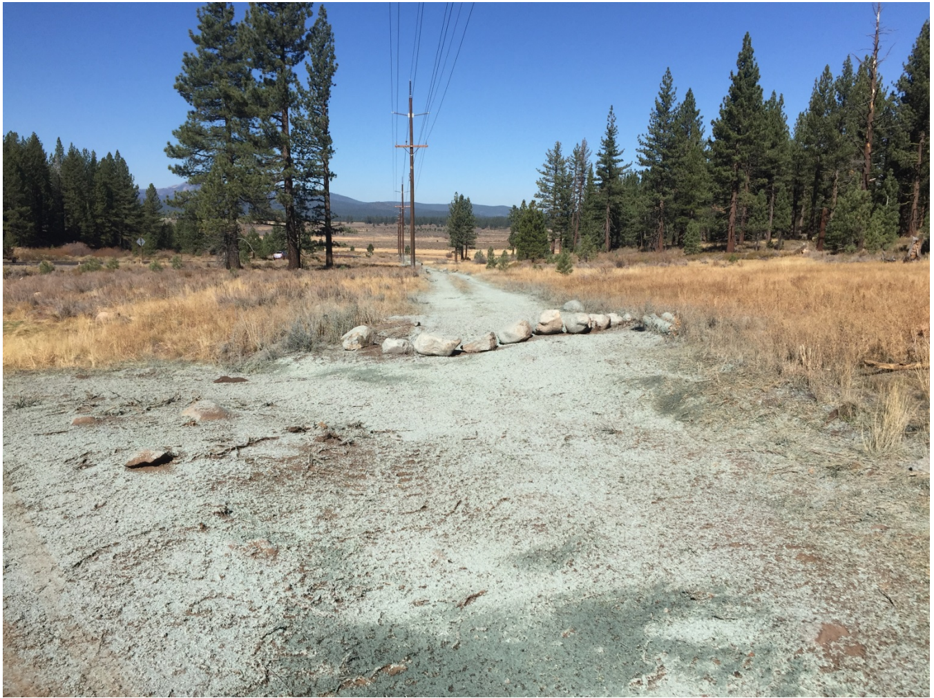
Photo 1: Right-of-way cleared of equipment and materials, rock barriers installed to prevent unauthorized access, and disturbed areas hydro-seeded. Between Poles #291080 and #291081.
