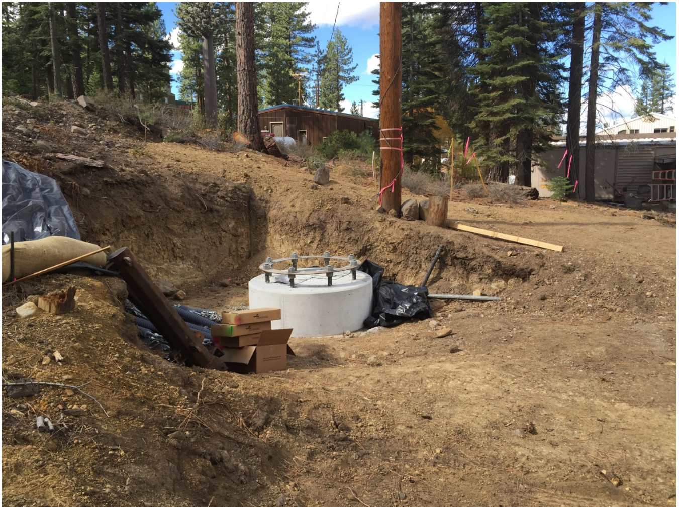
Photo 2: Base for Pole #291261 poured and being prepared for pole installation.
