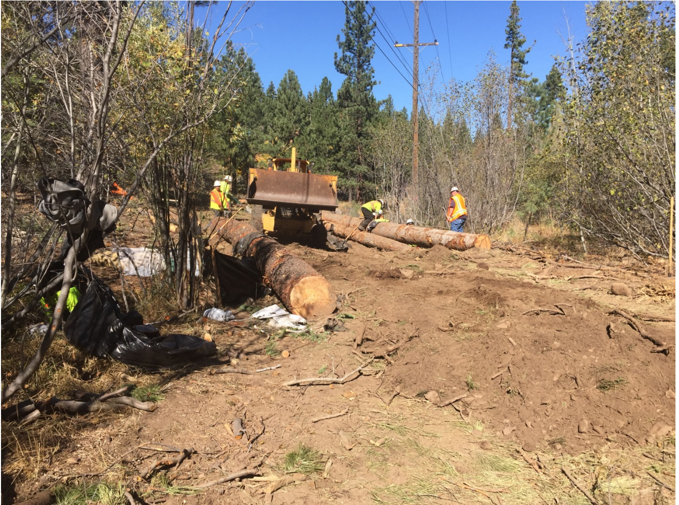
Photo 5: Spittler crossing at Pole #291110 being removed.
