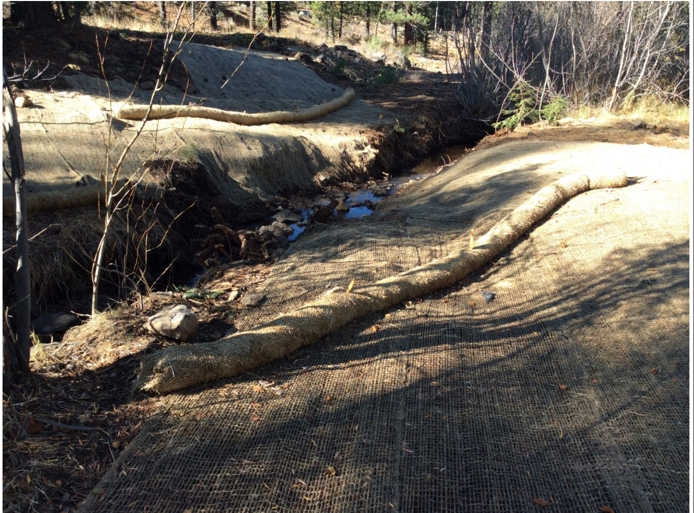
Photo 4: Spittler crossing near Pole #29110 removed and stream bank stabilized.
