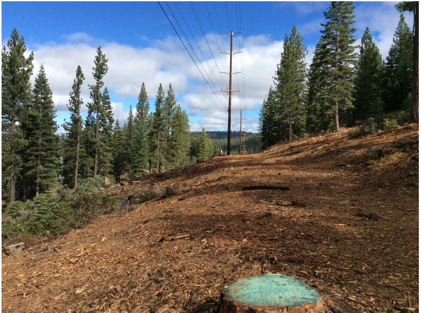
Photo 3: Restored and mulched ROW, cut stumps treated with borate compound per APM-BIO-4.
