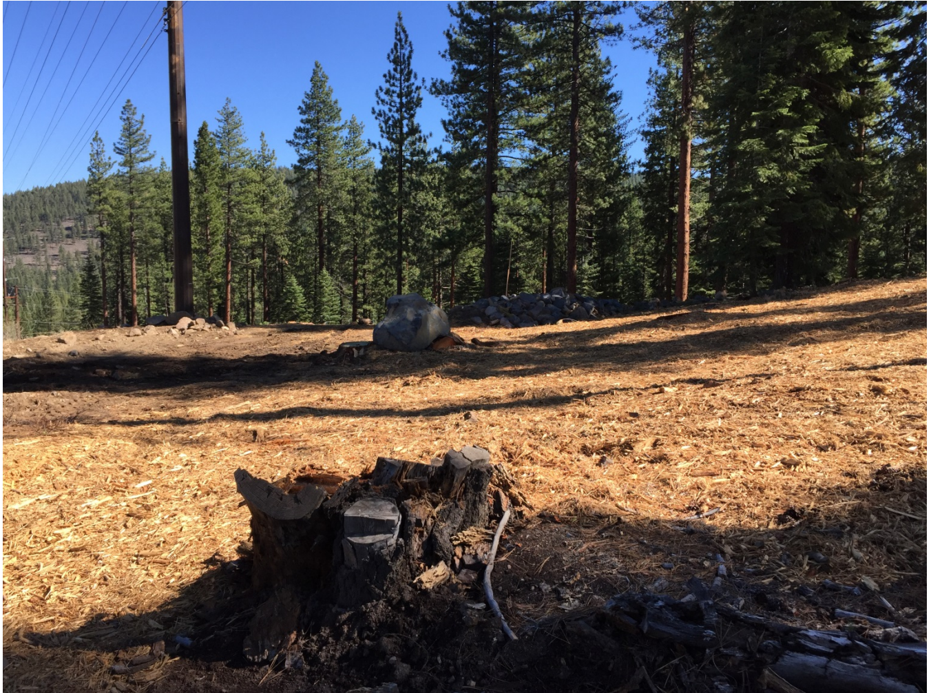
Photo 2: Mulch applied within disturbed areas of the new ROW along the Northstar fold, near Pole #291263.
