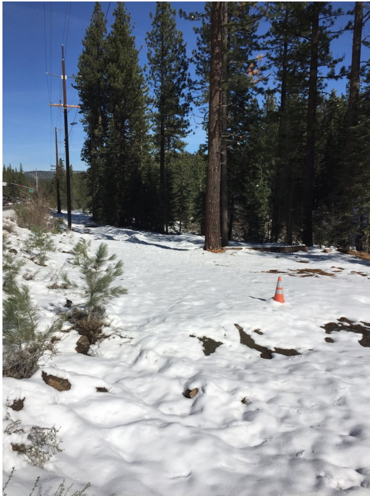
Photo 1: Looking north along Highway 267 toward Pole #291101 along ROW with snow on the ground. All work in this area has been completed (note, cone in ROW from CalTrans project work occurring on adjacent Highway 267).
