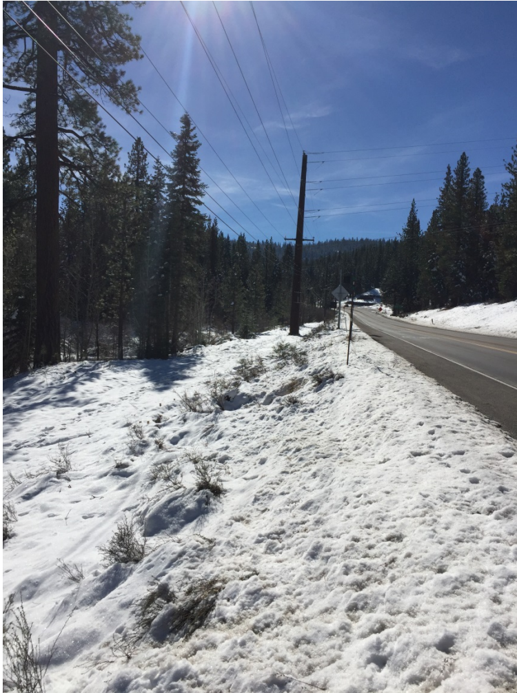
Photo 2: ROW along Highway 267, work completed.
