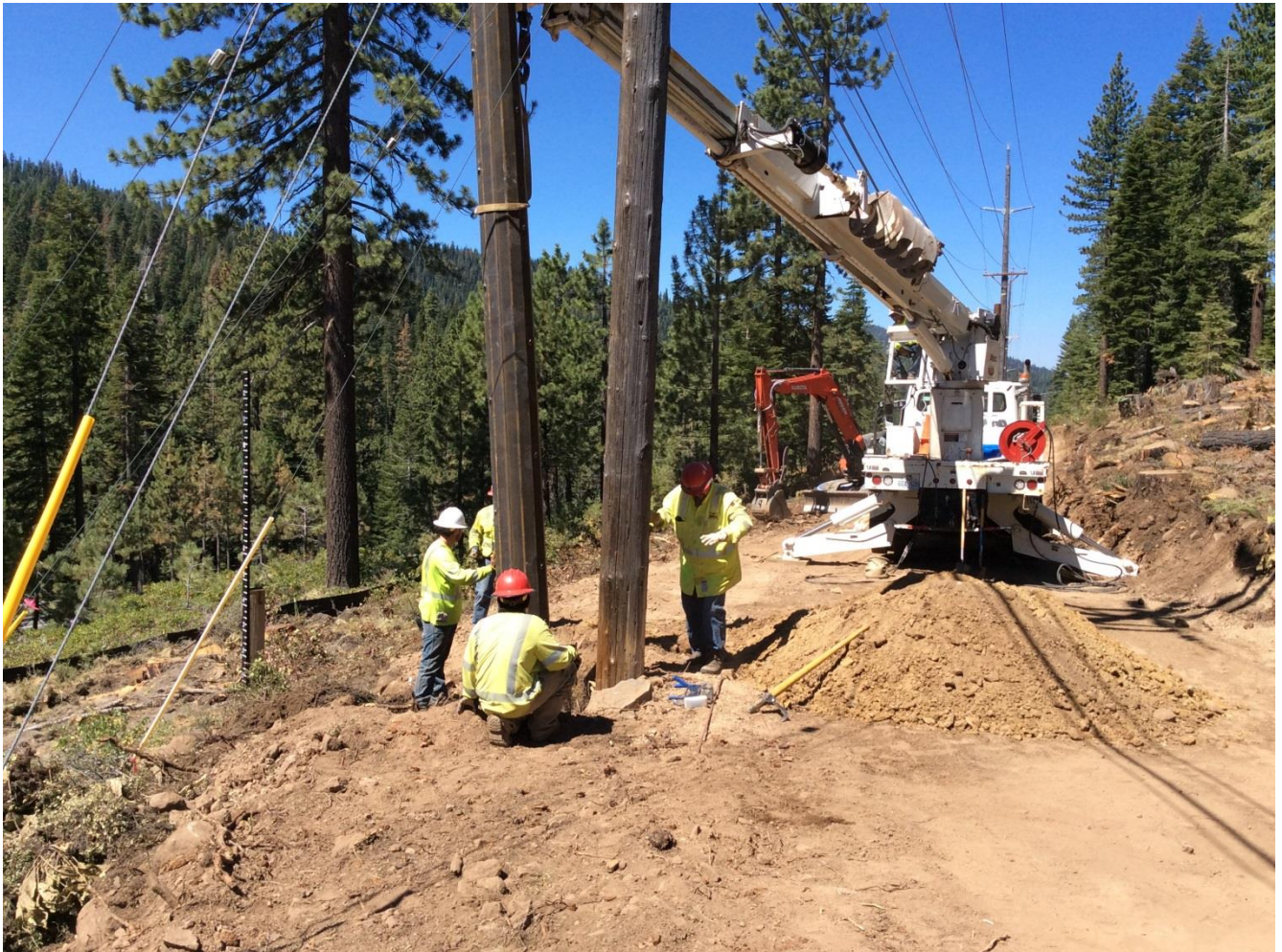
Photo 6: Crews installing angle Pole 291158.
