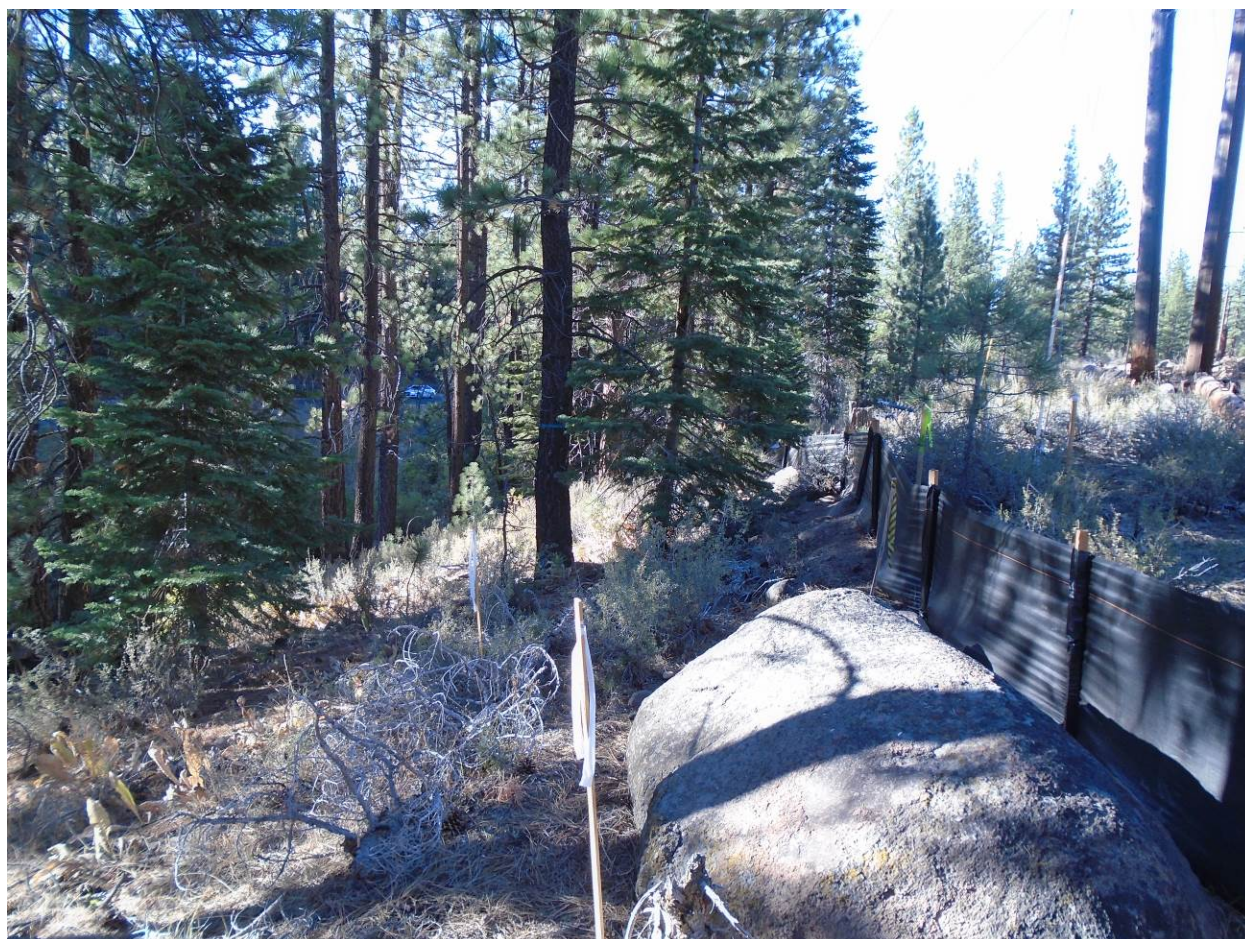
Photograph C-4: Pole 291087 Requested Additional Temporary Work Area Facing North
