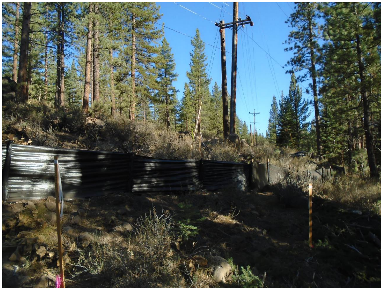
Photograph C-5: Pole 291087 Requested Additional Temporary Work Area Facing South
