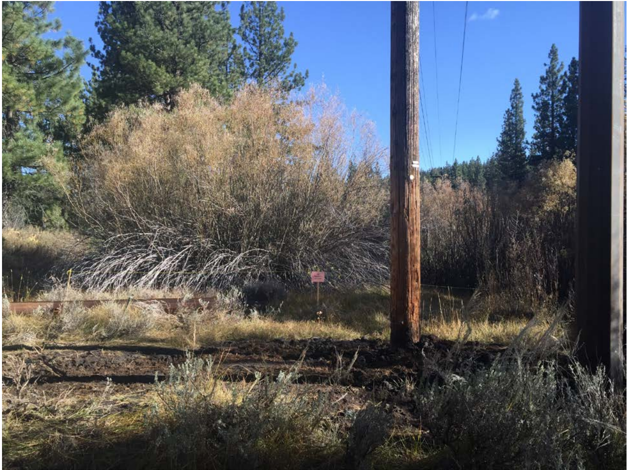
Photograph C-1: Pole 291098 Existing Workspace View Facing North
