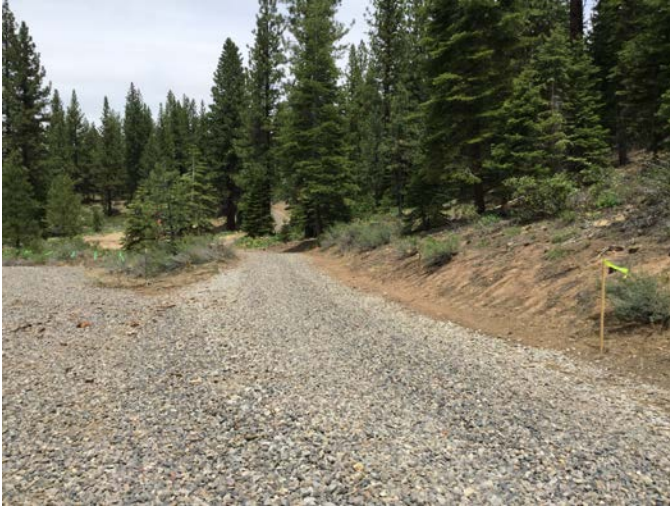
Photograph C-3: View of Existing Gravel Road Departing ROW at Pole 291110
