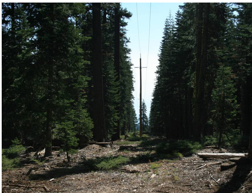
Photograph 14: An example of a permanent ROW, shown here along the existing 625 Line
