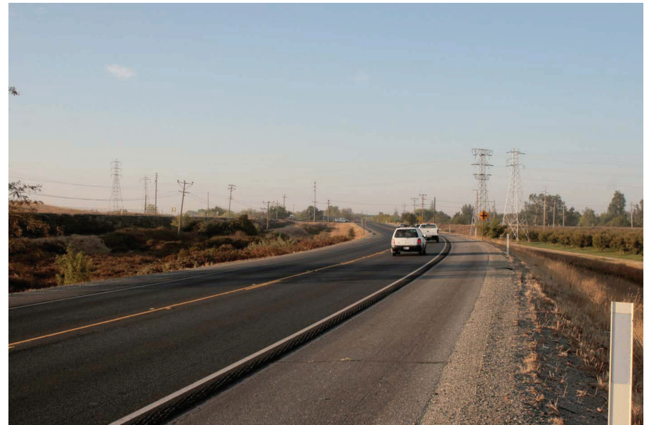
8. Highway 20 westbound looking southwest
