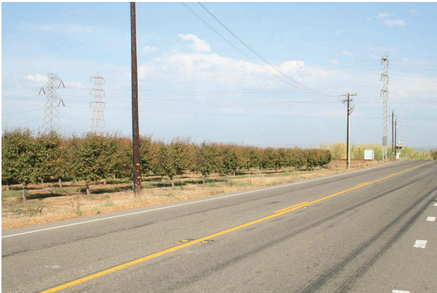
7. Ramirez Road east of Highway 70 looking east
