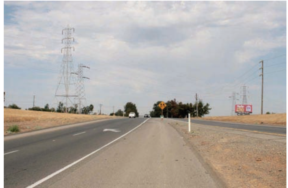
14. Highway 70 northbound at Highway 65 merge looking north*
