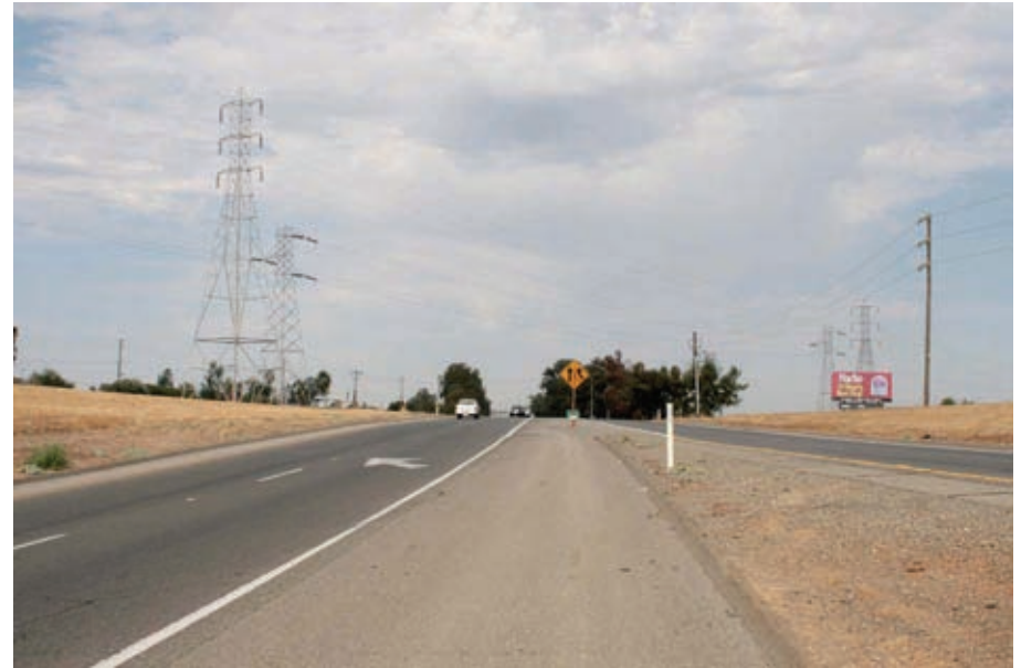
14. Highway 70 northbound at Highway 65 merge looking north*
