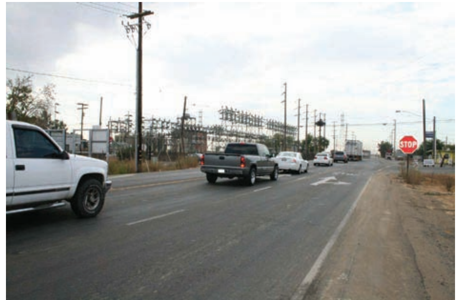
20. East Nicolaus Substation (from East Nicolaus Avenue and Highway 70)
