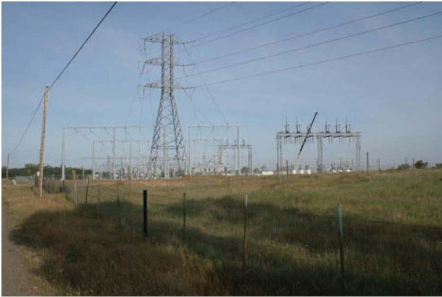
1. Stageline Road looking northwest toward Palermo Substation
