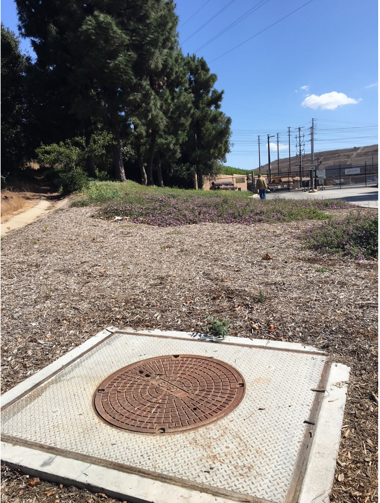
Photo 2. Looking south from V5022702 toward the nursery (behind the trees).
