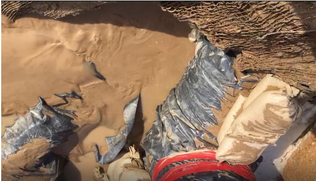
Photo 8: Water rapidly exiting the detention basin from area near the bottom of the standpipe following a large rain event. Water flowing under the plastic sheeting. Photo taken 1/18/2019.
