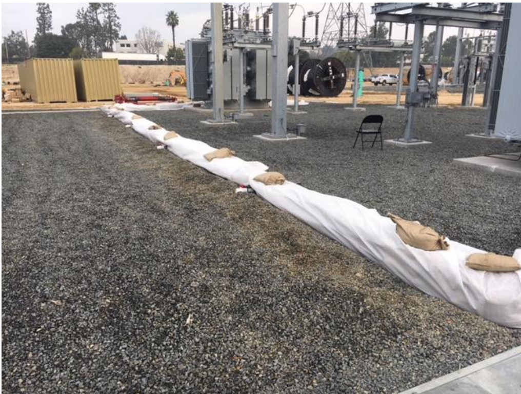
Photo 6 Temporary Containment Berms
