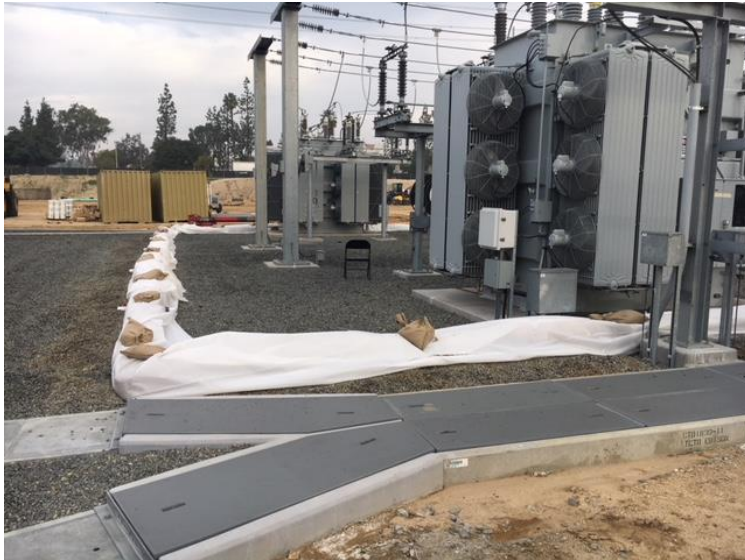
Photo 7 Temporary Containment Berms
