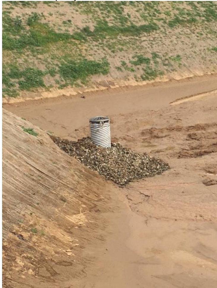
Photo 8 Gravel installed over sediment filter fabric at basin standpipe
