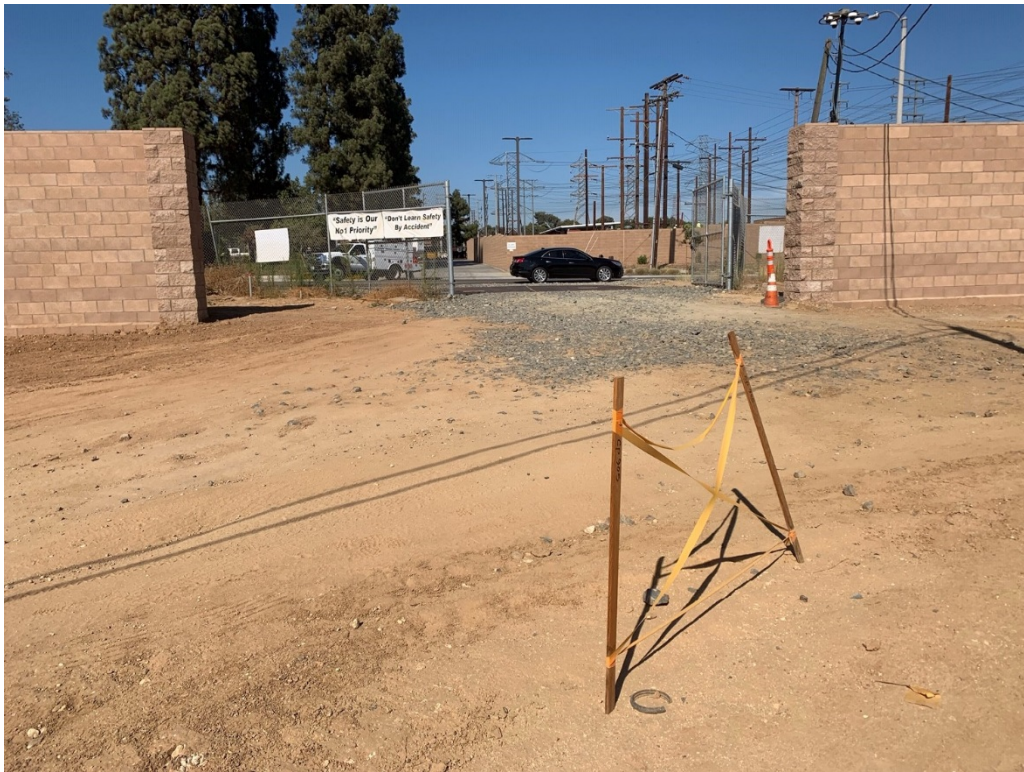
Photo 2. Looking ENE from M5701914 toward Marketplace Avenue.
