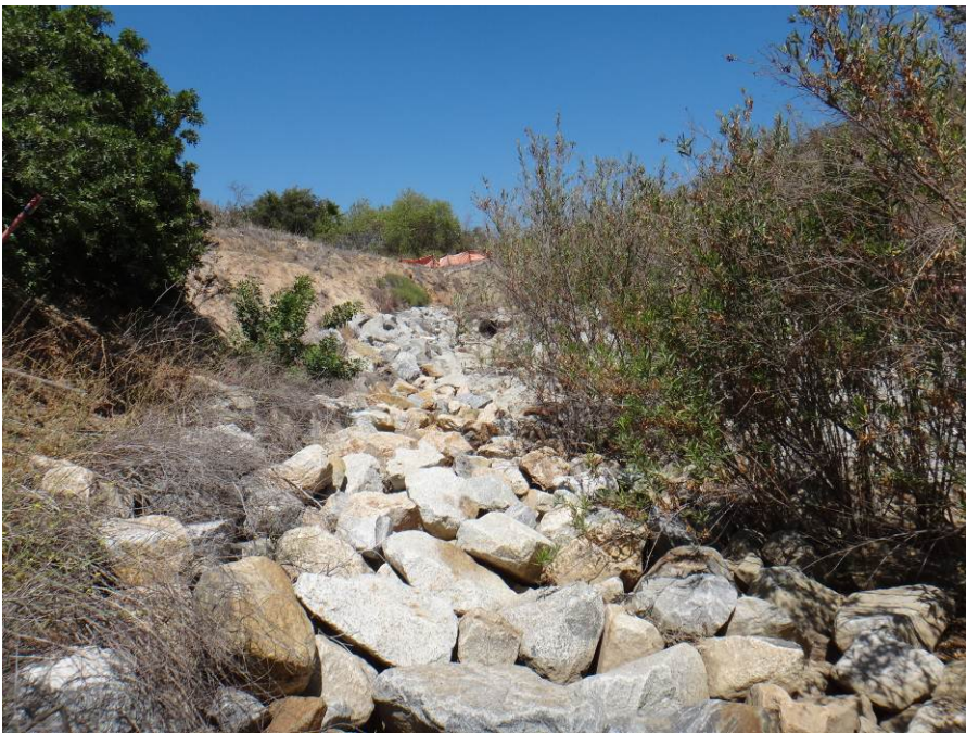
Photograph 22: Ephemeral drainage Feature 7-39-S-3, facing the culvert and upstream/east.
