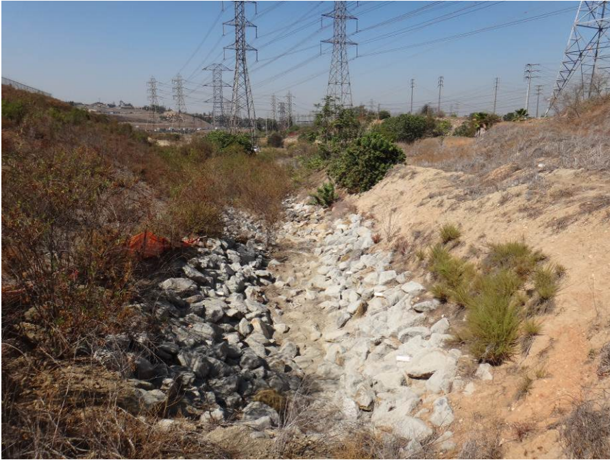
Photograph 21: Ephemeral drainage Feature 7-39-S-3, taken from above the culvert, facing downstream/west.
