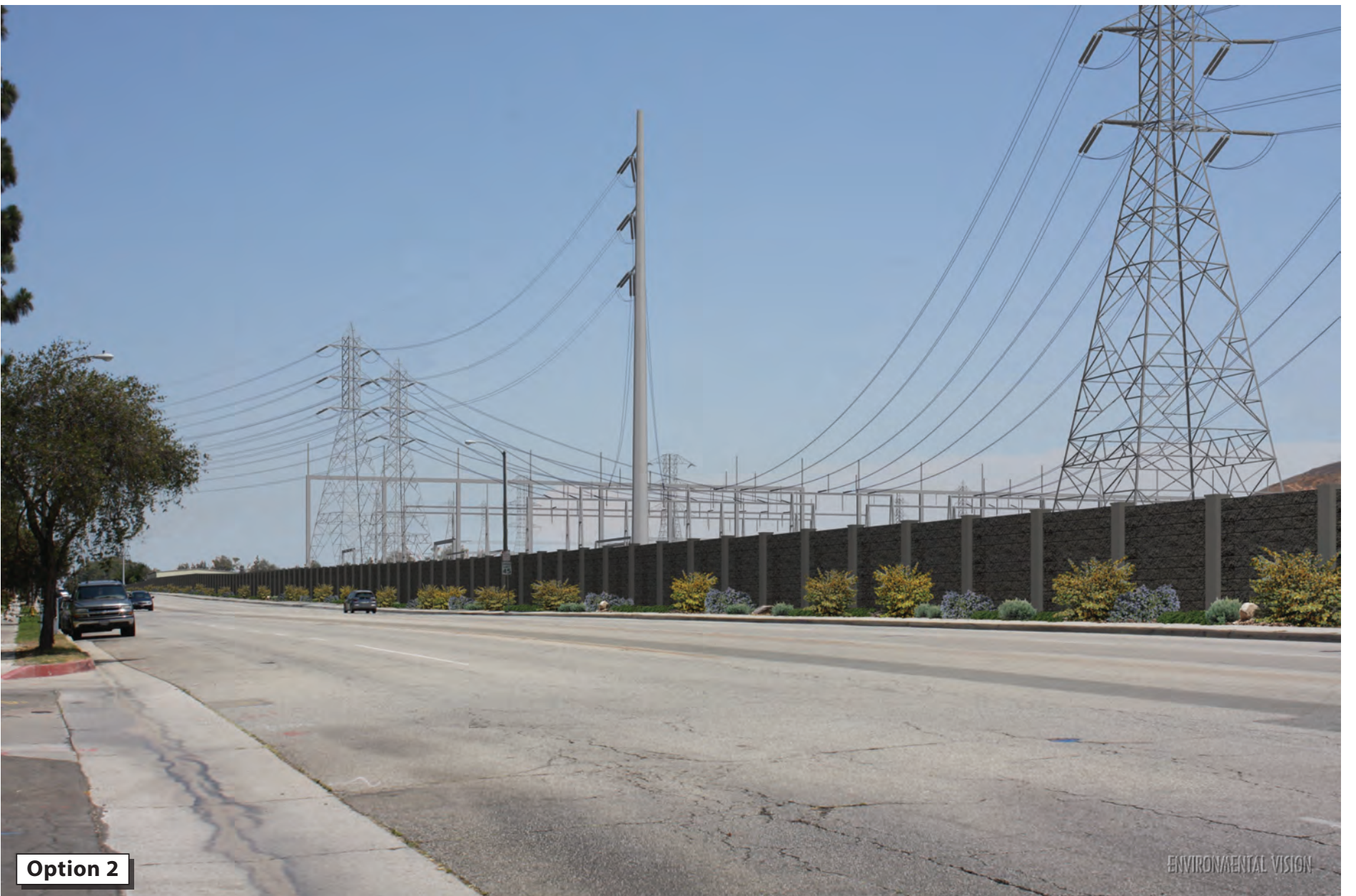
KOP 1 – Visual simulation of the Proposed Project with shrub and groundcover landscaping
