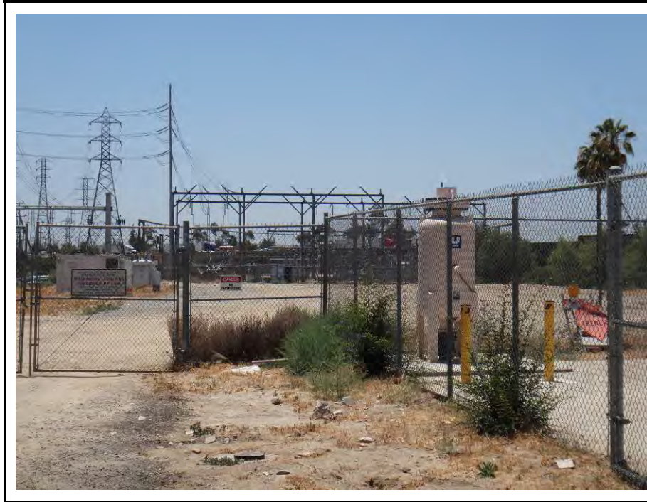
Photograph 15: Representative photograph of disturbed/developed habitat at the Goodrich Substation site.
