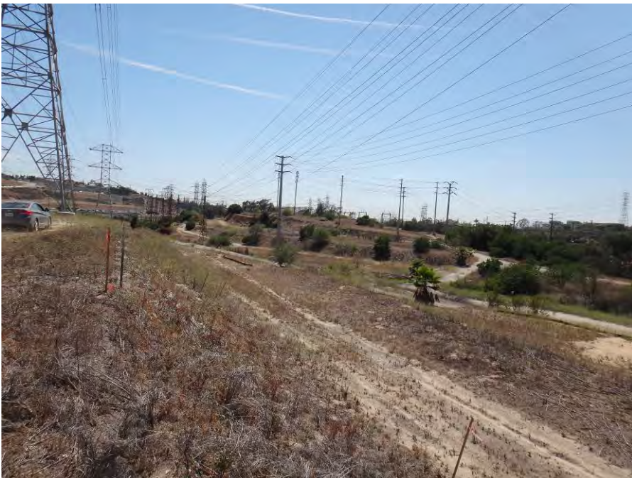
Photograph 6: Representative photograph of ruderal grassland and disturbed/developed habitat at the Mesa Substation site.
