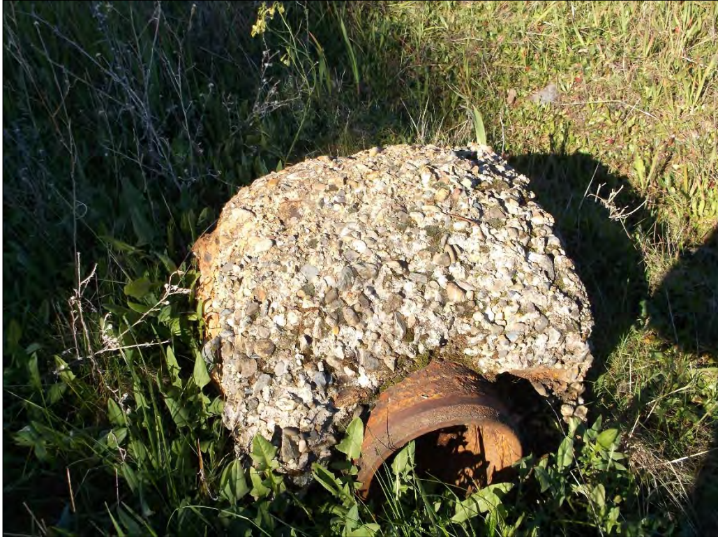
Photo 10. IO 1. Aggregate concrete/metal culvert.
