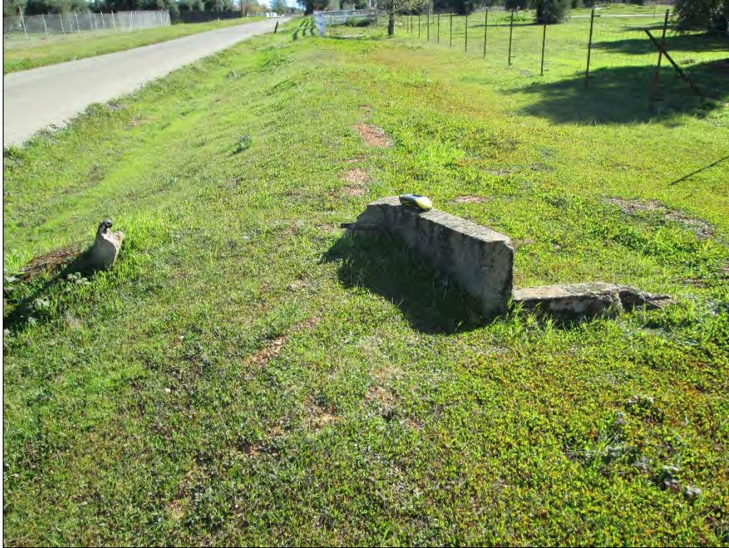
Photo 14. IO 10. Concrete structure.
