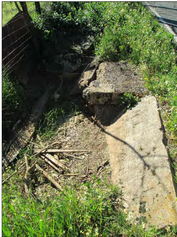
Photo 18. Concrete-lined portion of Happy Valley Ditch.
