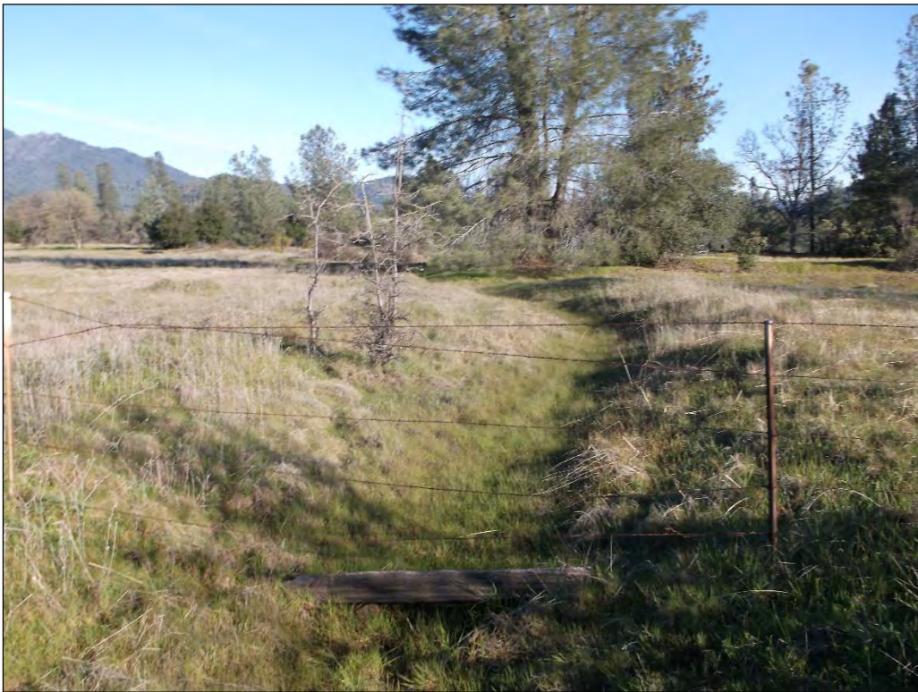
Photo 16. Happy Valley Ditch, crossing Cloverdale Road. View is to the north.
