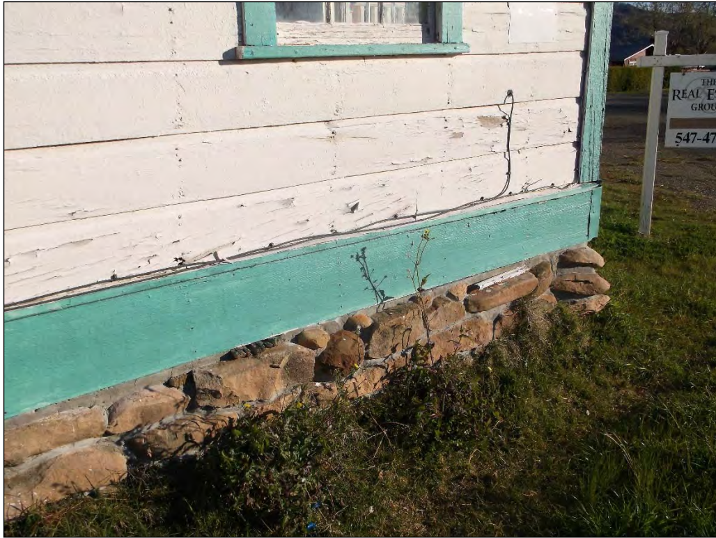
Photo 22. Igo Inn, detail of northeast foundation corner.
