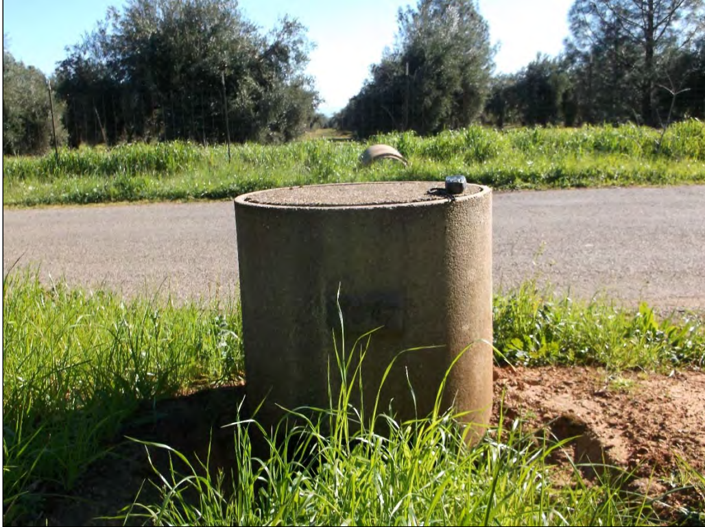
Photo 12. IO 4. Concrete pipe with 1942 inscription.
