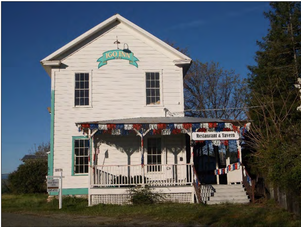
Photo 20. Igo Inn, front. View is to the southwest.
