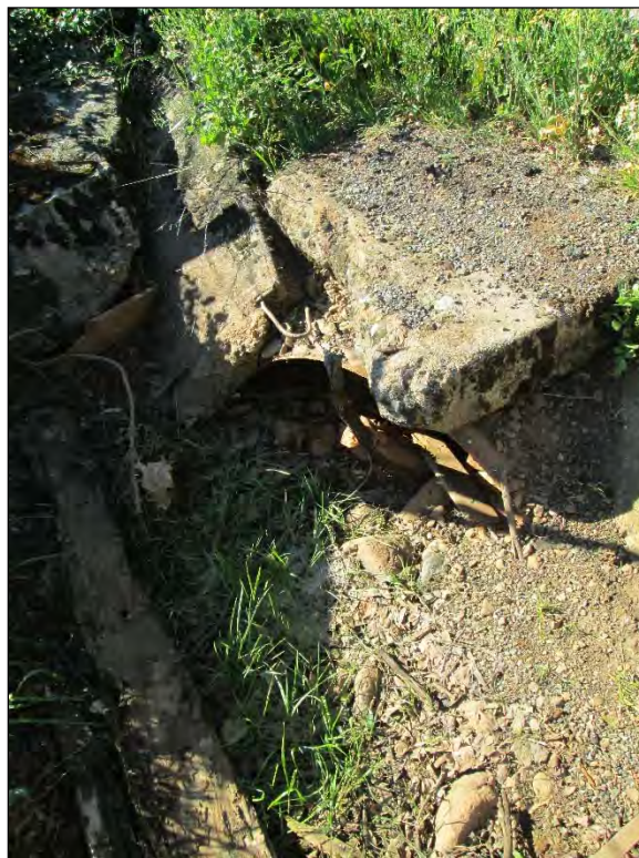
Photo 19. Concrete-lined portion of Happy Valley Ditch.
