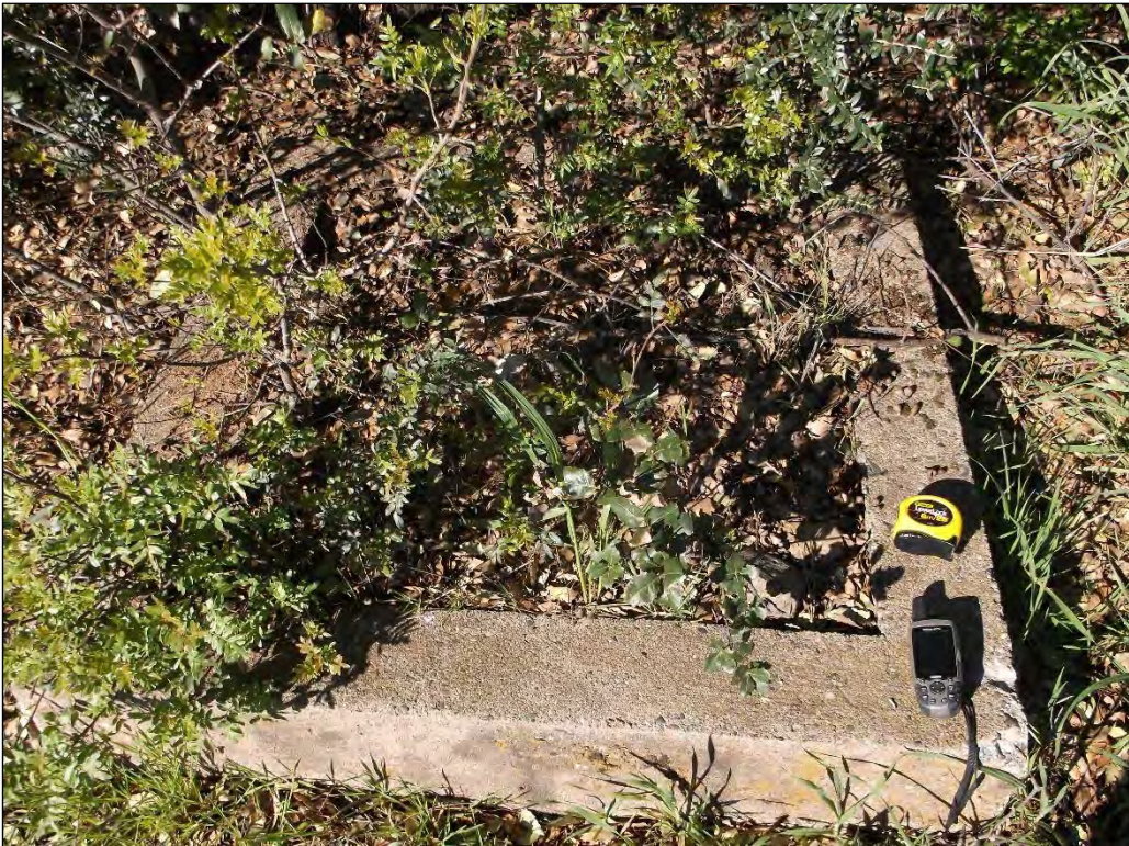
Photo 11. IO 3. Concrete "box."
