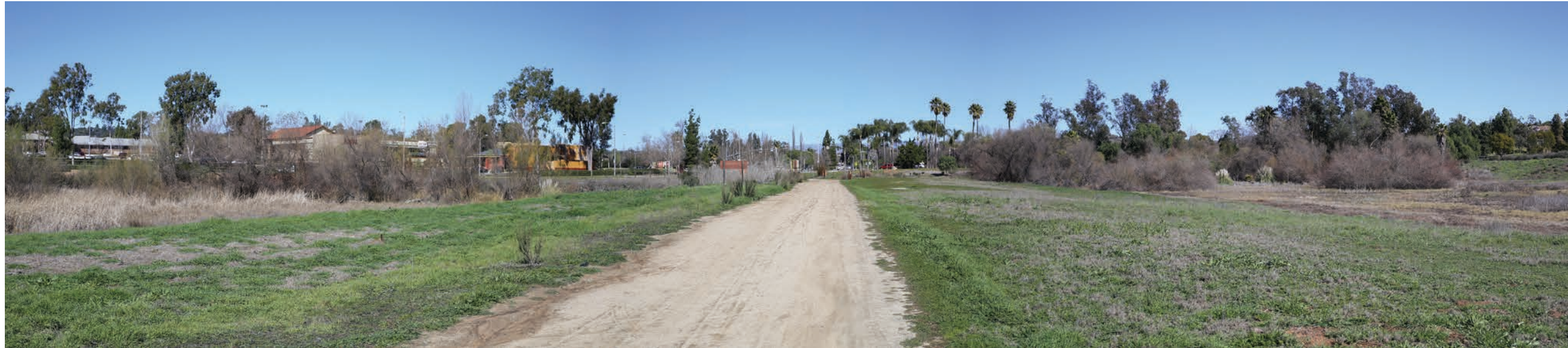
Existing view looking north along Mule Hill Trail near approximate MP 29.4, where the proposed MLV 7 and Line 1600 Cross-tie structure will be located.
