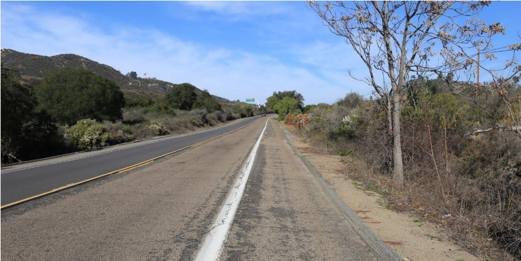
Photograph 21: View looking north-northwest toward the location of MLV 5 along North Centre City Parkway near approximate MP 20.1. The MLV is depicted by the red box. Small- and medium-sized shrubs within the workspace are expected to be removed at this location. The remaining shrubs to the north and south of the MLV that are outside of the workspace will limit views of the MLV.
