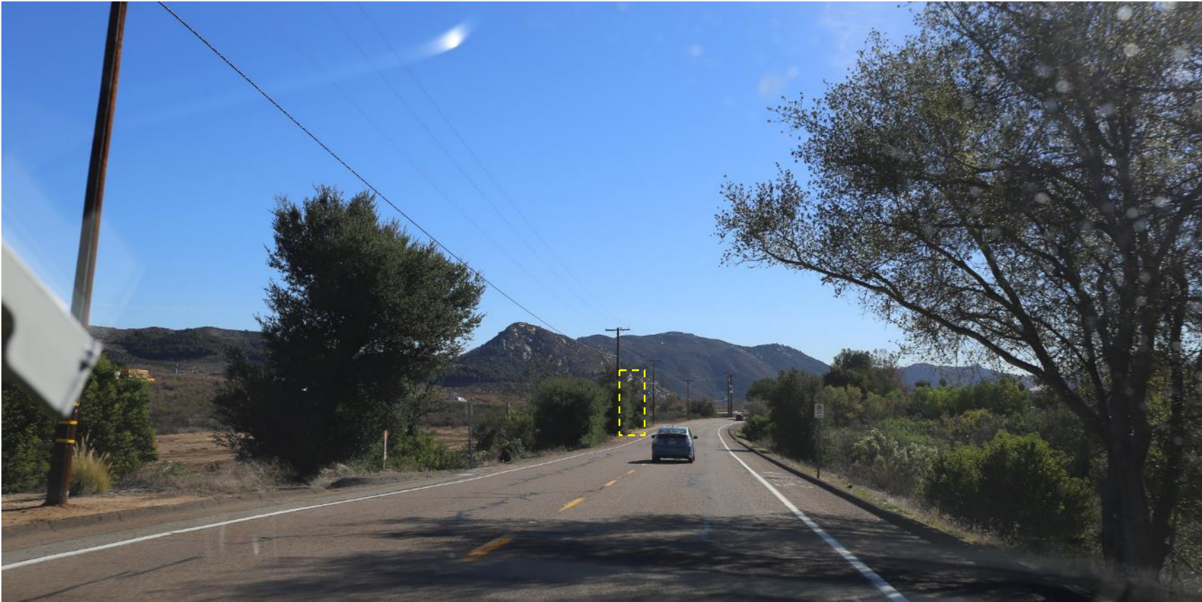
Photograph 10: The location of proposed MLV 2, looking south-southwest along Old Highway 395 near approximate MP 6.2. The yellow box depicts vegetation removal that will likely be required for workspace during construction. As discussed for Photograph 9, the MLV location is set slightly below the road level, which limits its visibility from a distance. In addition, the MLV will be largely obscured from this direction due to foreground vegetation that will not be removed for the Proposed Project.
