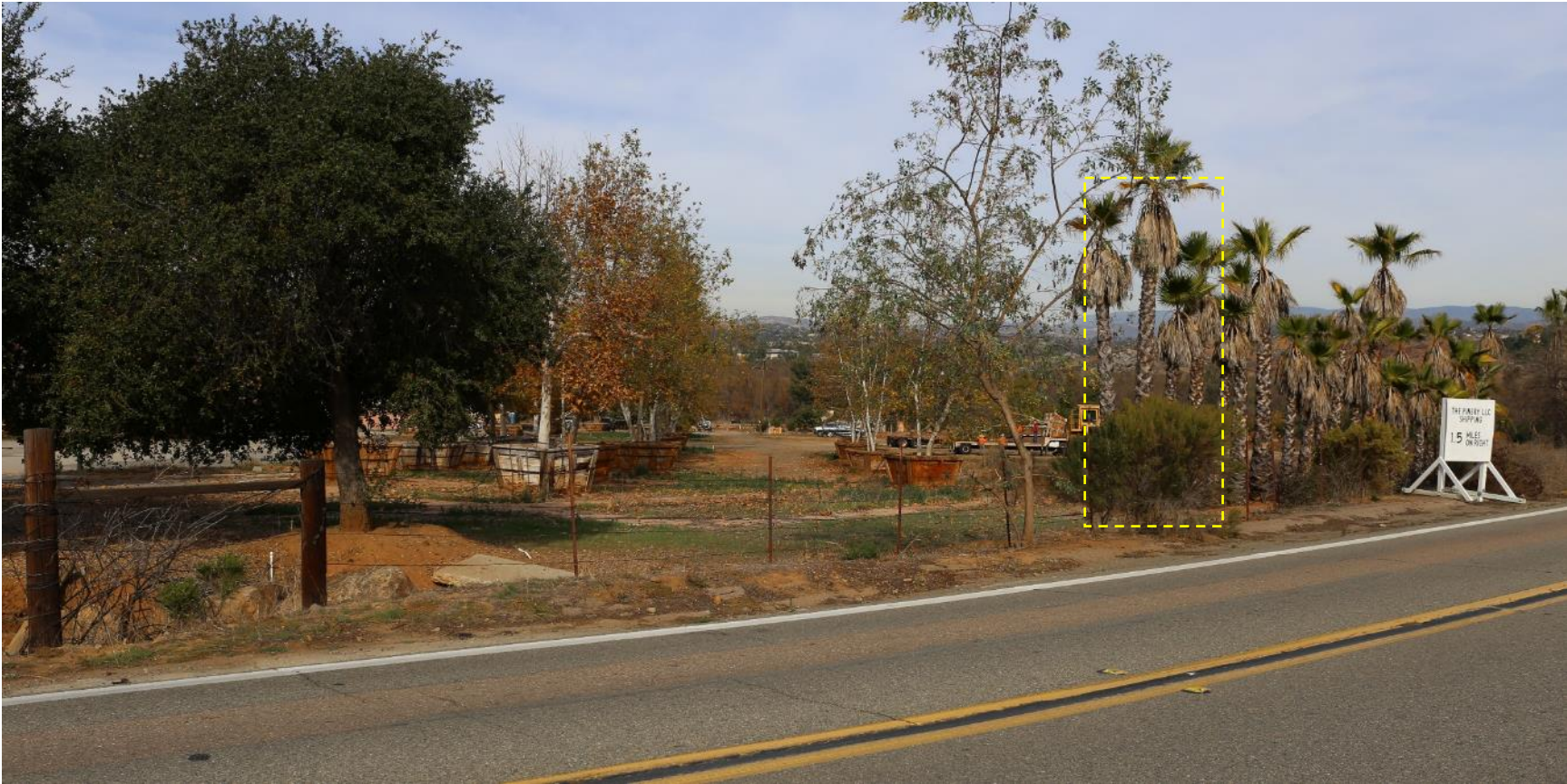
Photograph 29: View looking north along Highland Valley Road toward the Lake Hodges HDD workspace near approximate MP 30.5. Minimal vegetation disturbance is expected to occur here as most of the plants are potted. The vegetation anticipated to be removed is depicted by the yellow box in the photograph. The roadside vegetation is not anticipated to be removed, and will partially obscure the disturbance from vehicles.
