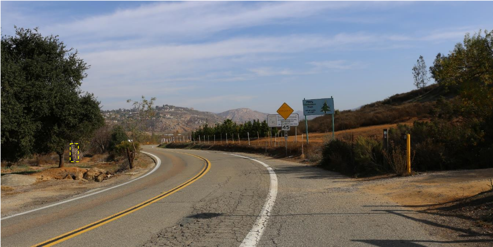
Photograph 28: View looking east along the east-bound lane of Highland Valley Road near MP 30.5. Minimal vegetation disturbance is expected to occur in this location as a result of the Lake Hodges HDD workspace because most of the plants are potted (much of the area is utilized as a large tree nursery). The yellow box depicts the potential vegetation removal area. Views from vehicles traveling along the road will be generally obscured by the surrounding vegetation that will not be removed.
