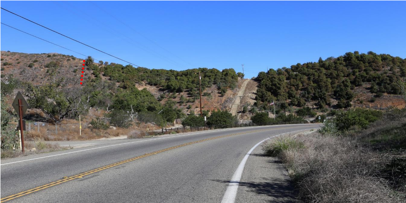
Photograph 6: View looking northeast from Mission Road of the Proposed Project ROW near approximate MP 3.9. The ROW, which is depicted by the red line, will only be visible for a short period of time while driving along Mission Road. The view of the alignment is limited by trees in the foreground and the road turning away from the site.
