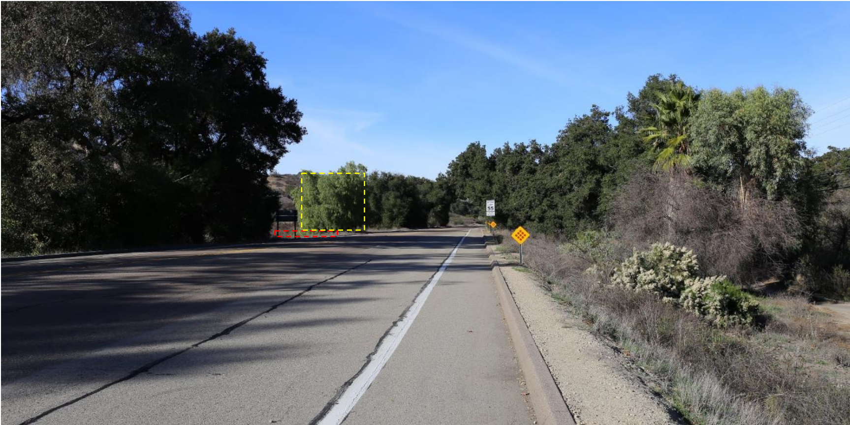
Photograph 18: View looking north-northwest toward the location of MLV 4, along Old Highway 395 near approximate MP 15.5. The MLV is depicted by the red box, and the potential vegetation removal is depicted by the yellow box. Most of the surrounding large trees are not expected to be removed during construction. The vegetation will generally block views of the MLV from vehicles traveling in either direction until directly adjacent to the MLV. Additionally, the proposed site is set approximately five feet below the road level, which partially obscures views of the MLV.
