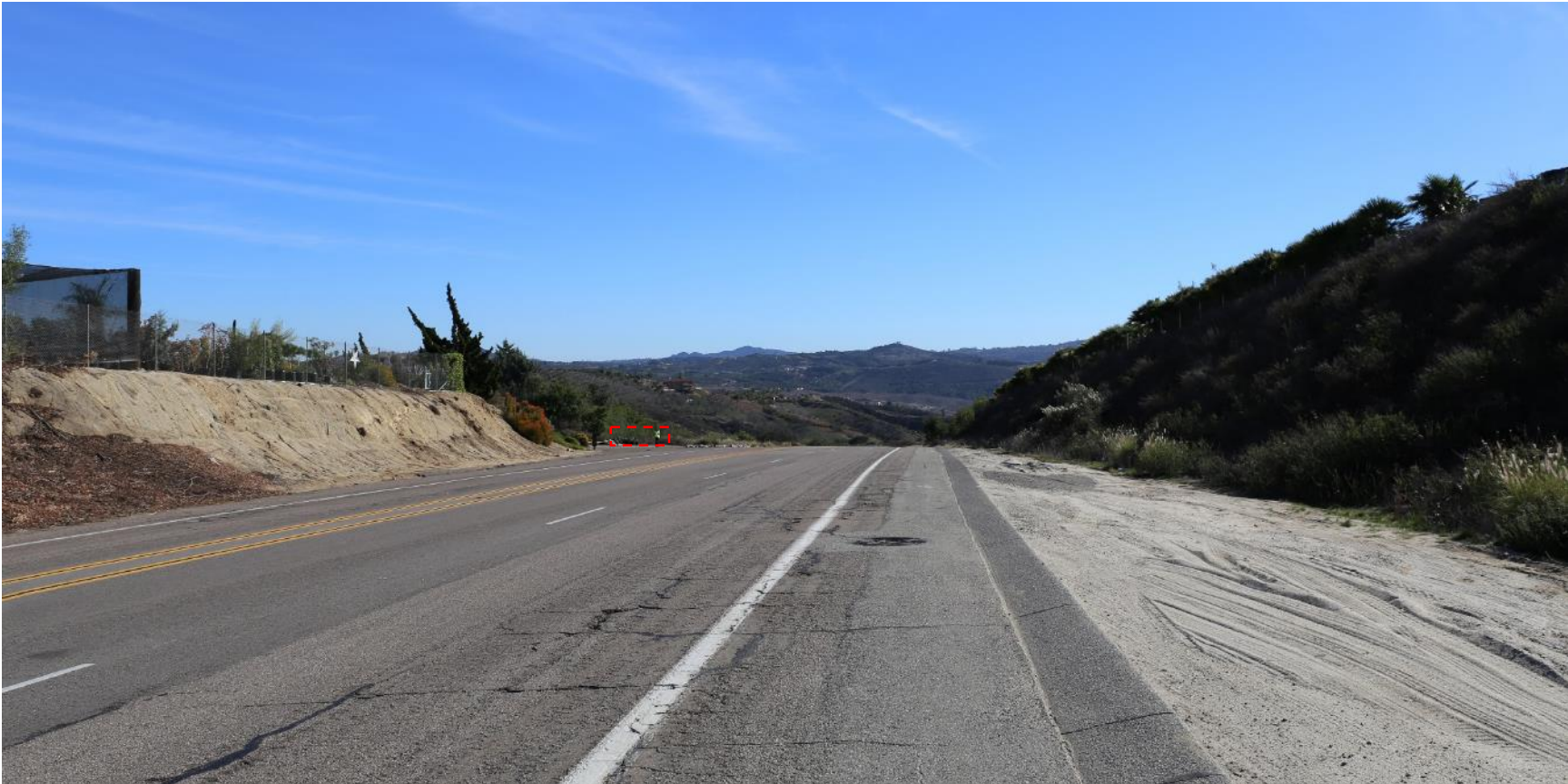
Photograph 12: View looking southeast toward the location of proposed MLV 3, along Old Highway 395 near approximate MP 10.8. No vegetation removal is anticipated at this location. The MLV is depicted by the red box, and is generally visible by vehicles traveling along Old Highway 395.
