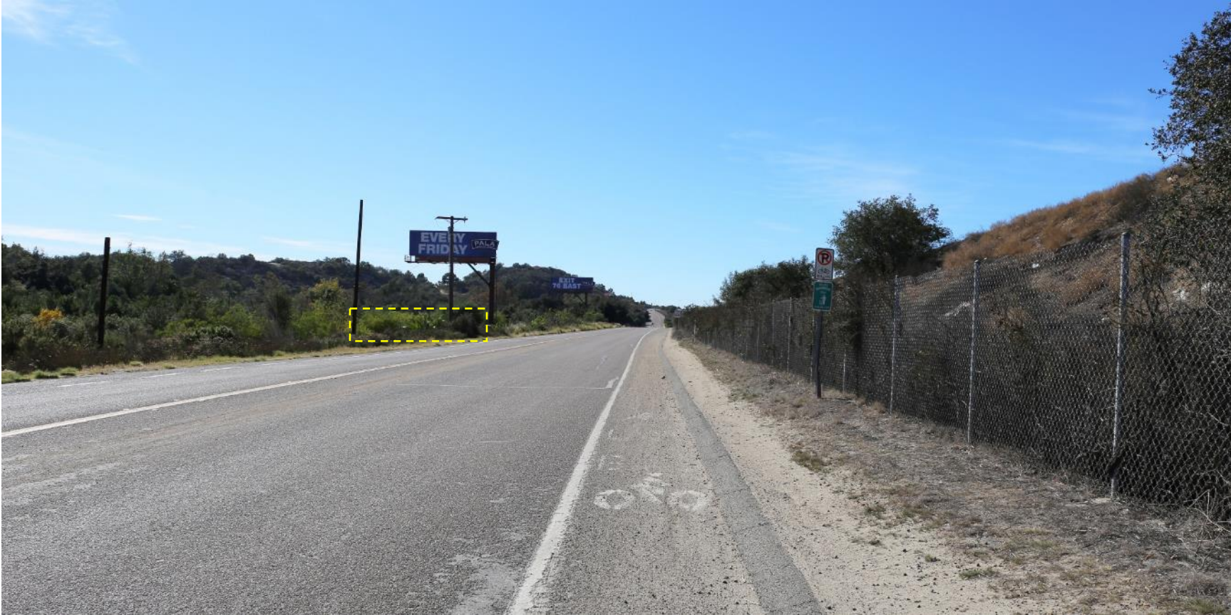
Photograph 1: View looking south along Old Highway 395 at approximate Milepost (MP) 1.5. The MLV 1 walls will most likely not be visible from Interstate (I-) 15 due to the approximately 10-foot drop off the side of the roadway, which is shown in Photograph 2. Minor vegetation removal will be required at the location indicated by the yellow rectangle. The area is visible only to passing cars traveling along Old Highway 395 when directly adjacent to the location, and most vegetation in the area is potted ornamental plants.
