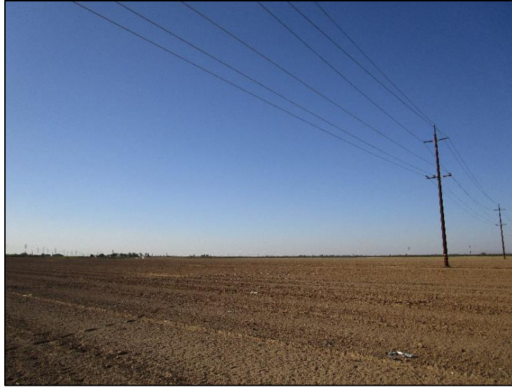
Photo 2. View facing northwest of Sanger Substation. 36.707235, -119.612191.
