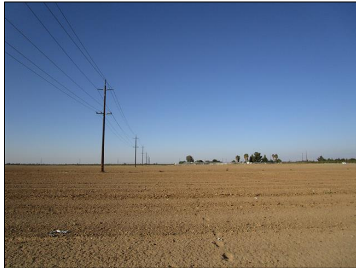
Photo 3. View facing north, west of Sanger Substation within the temporary staging area. 36.707959, -119.612207.
