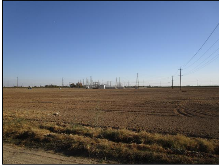
Photo 5. View facing southeast from the canal northwest of Sanger Substation. 36.710208, -119.612182.
