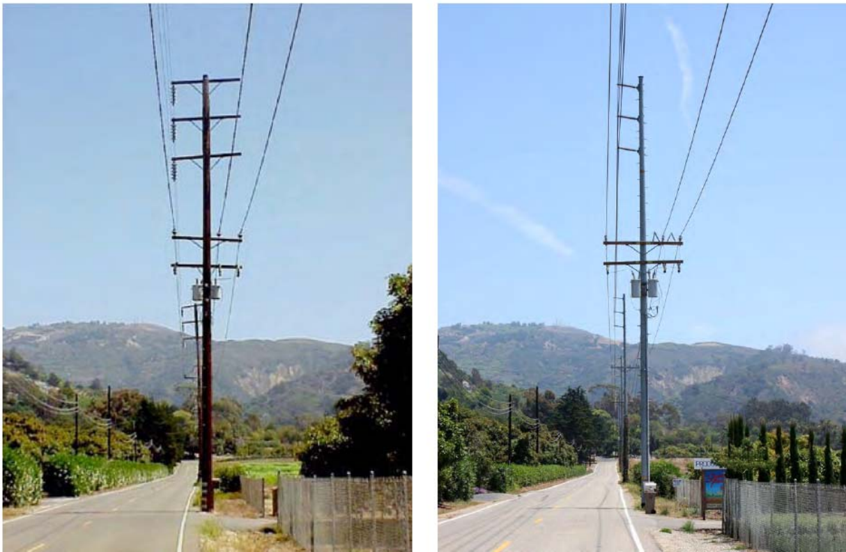
Left to right: On the left, pre-2004 wooden poles; On the right, post-2004 LWS poles
