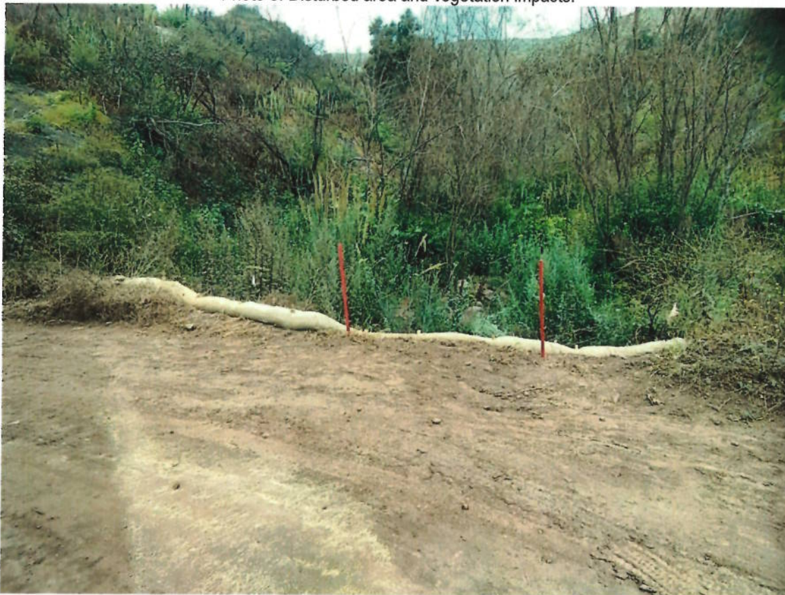
Photo 4: Straw wattles were installed after the area was stabilized.
