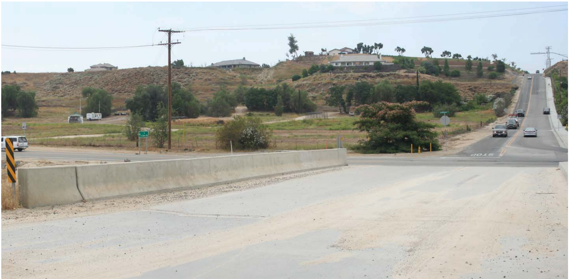
a. KOP 1 - Existing view of the Triton Substation site looking southeast from Liefer Road at a point immediately north of the intersection with Nicolas Road.
