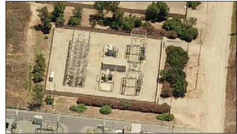
Border Substation (Pictometry.com 12/24/2014)
