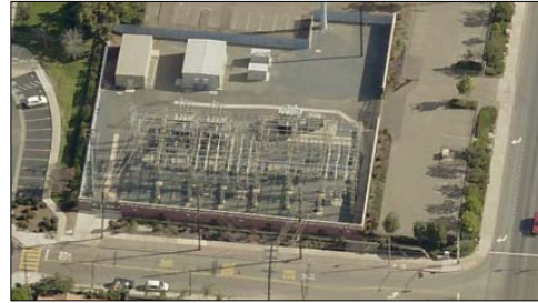
Otay Substation (Pictometry.com 12/24/2014)
