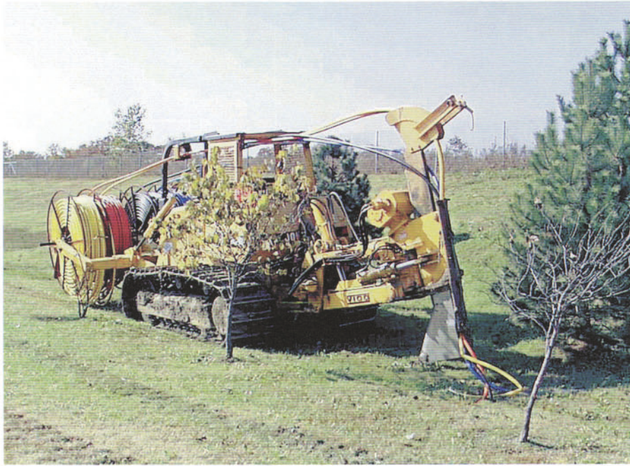
Cable installation using plow
