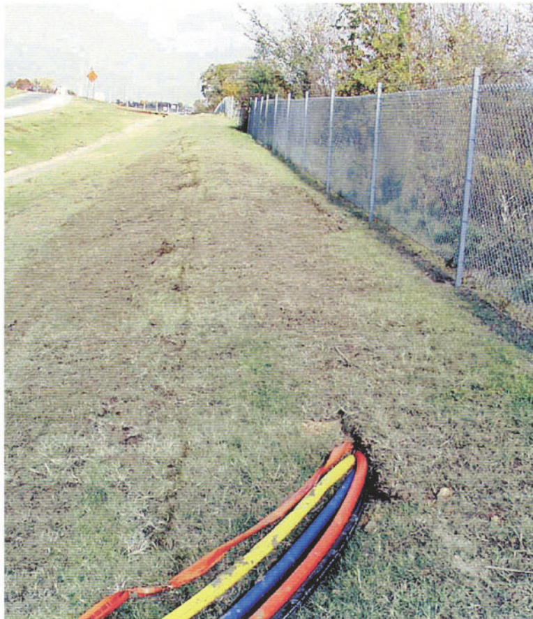
Site after installation using plow
