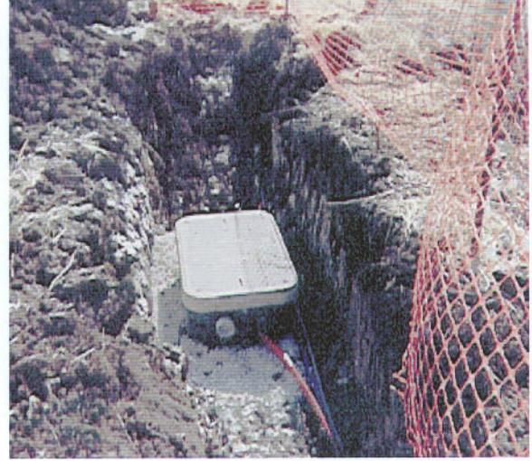
Handhole Installation
