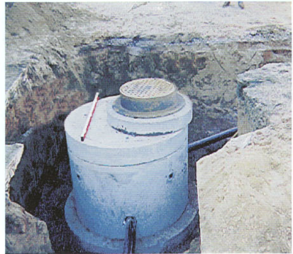
Manhole Installation
