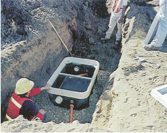
Handhole Installation
