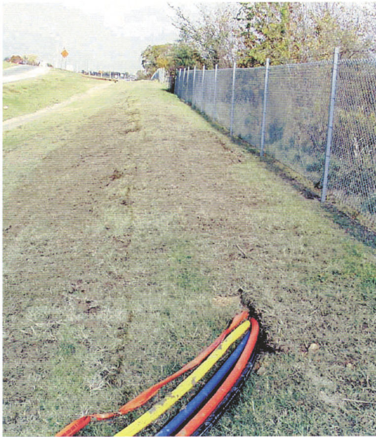
Site after installation using plow
