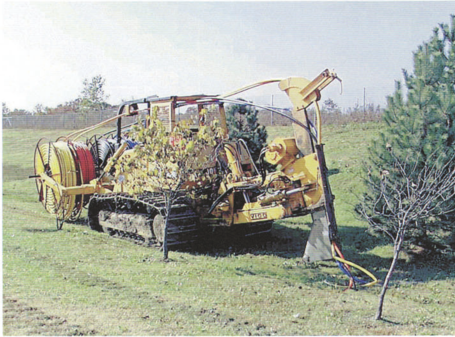
Cable installation using plow
