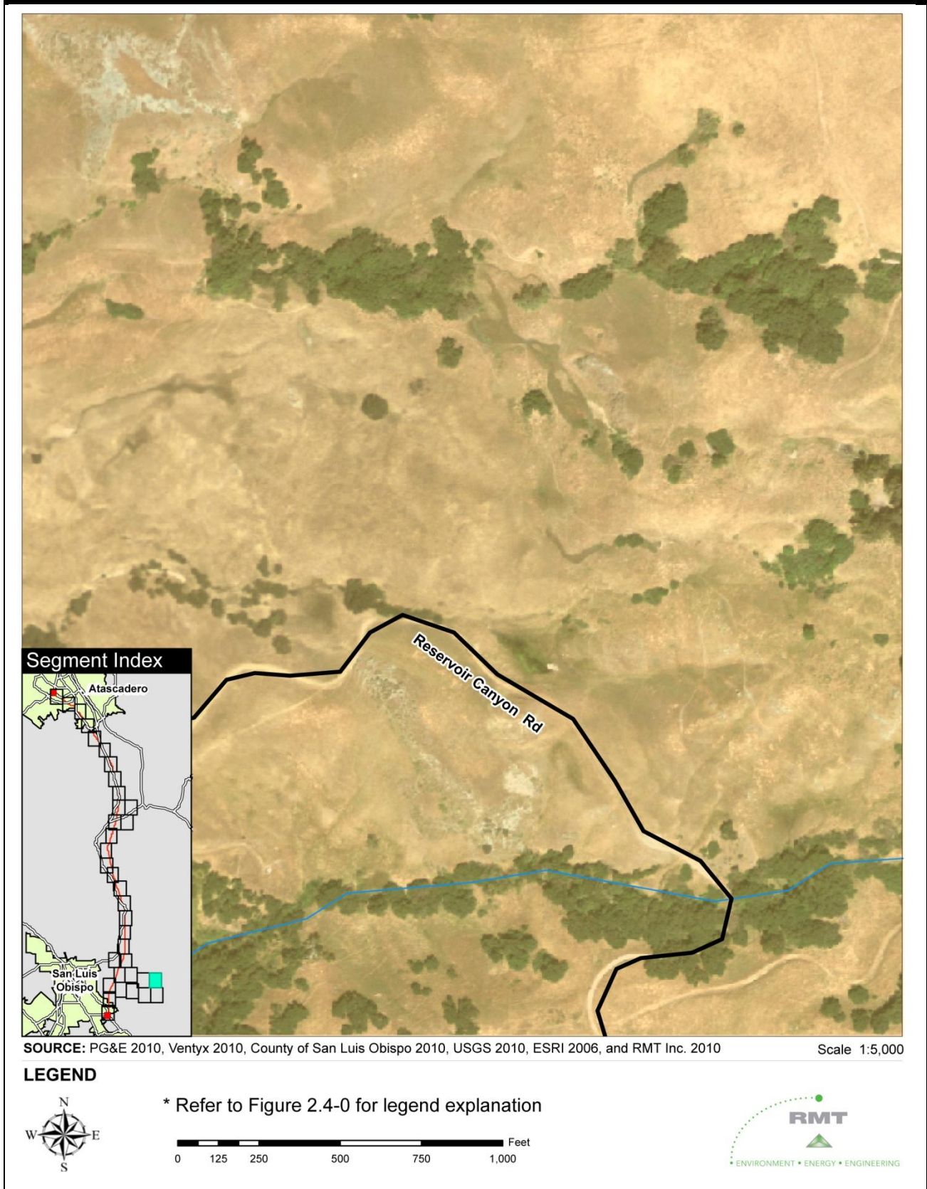
Figure A-31: Power Line Segment (31 of 35)
