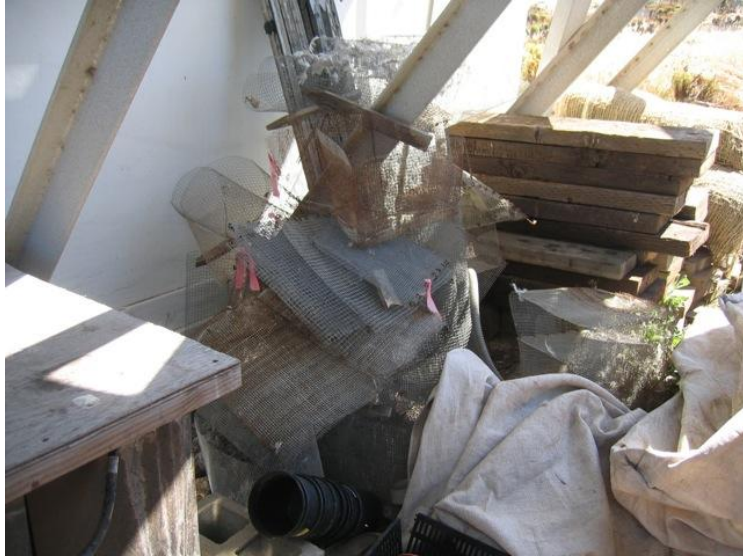
Figure 25 – Anacapa location for our batteries
