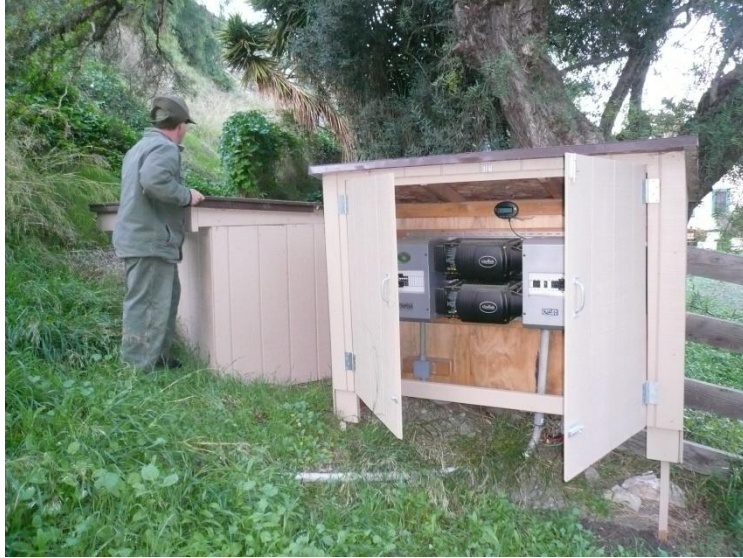
Figure 8 – Existing shed/cabinet at Scorpion
