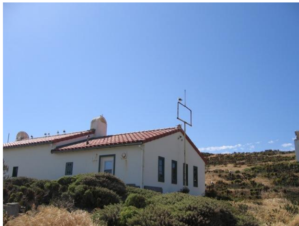
Figure 20 – Anacapa Generator Building Lat 34° 00' 55.73" N, Long 119° 21' 48.14" W
