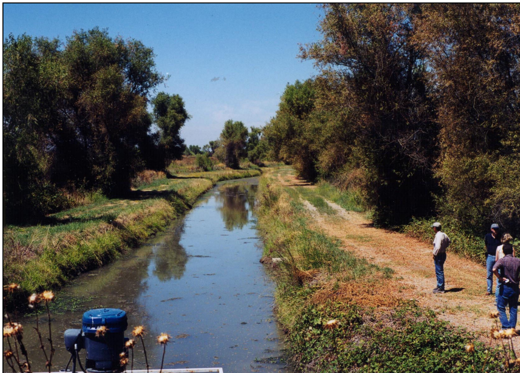
Figure 3.1-2: Storage Loop Pipeline Visual Setting
