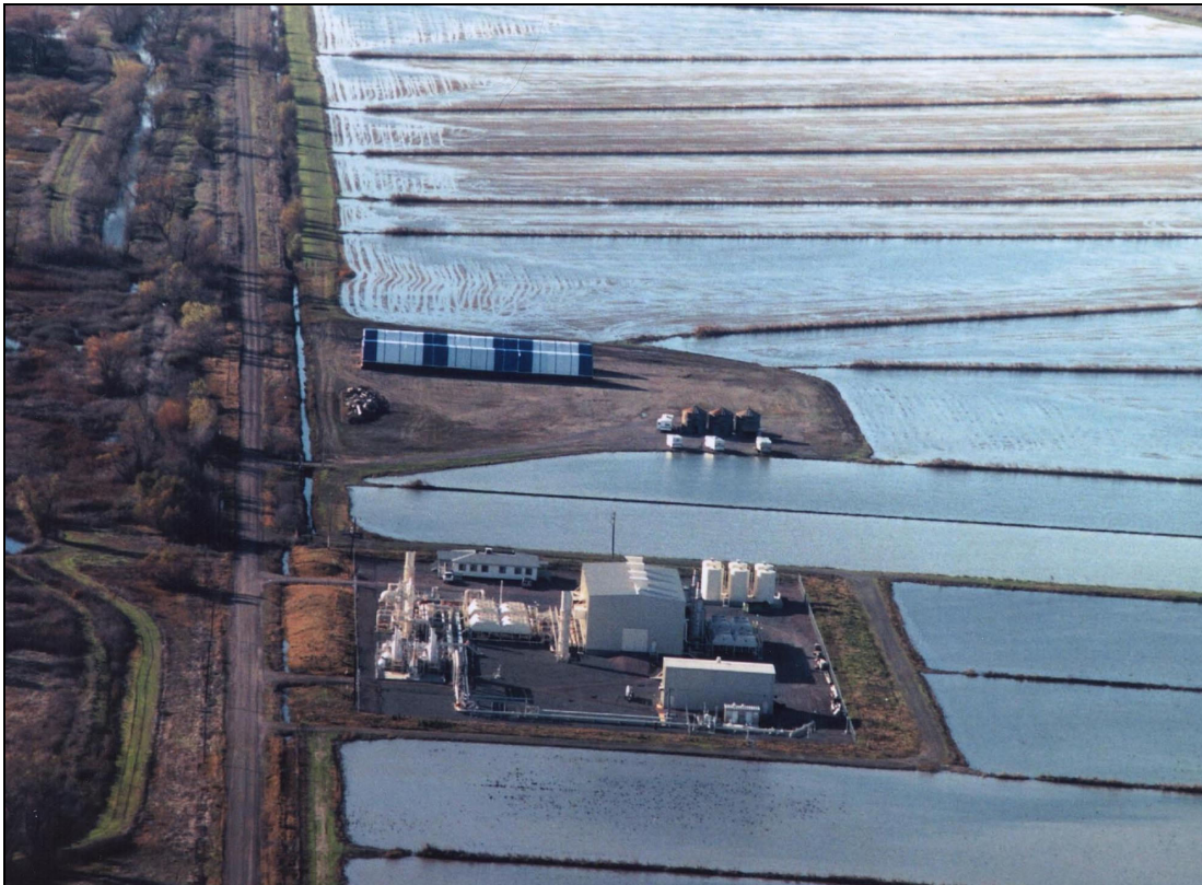
Figure 3.1-3: Remote Facility Site Visual Setting with Adjacent Rice Fields
