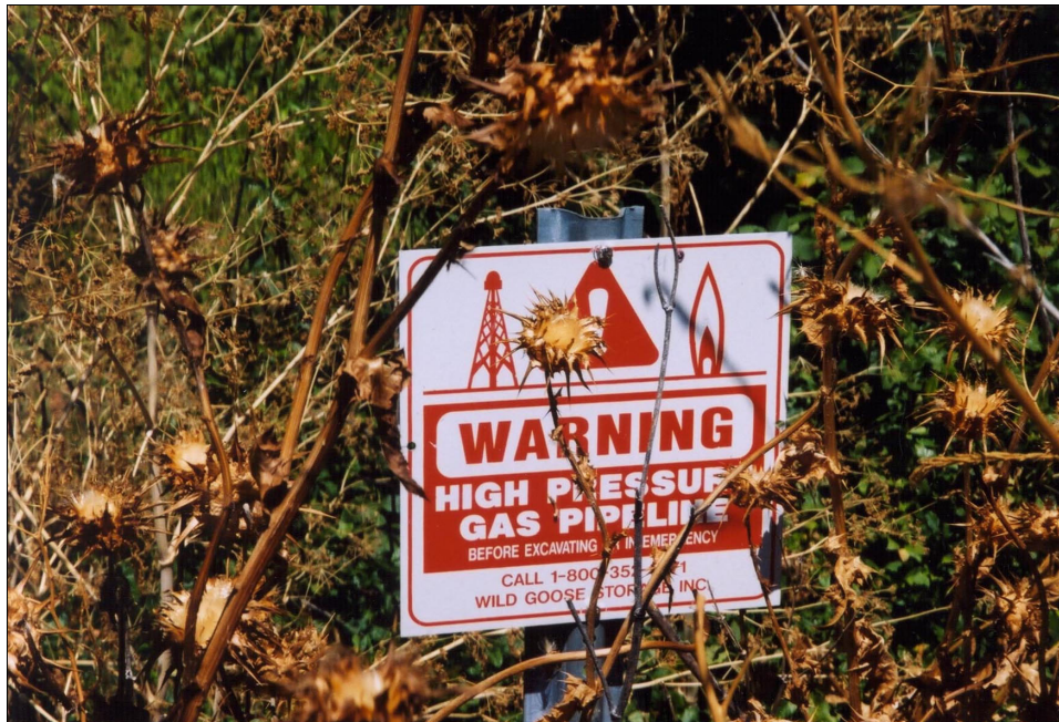
Figure 3.1-5: Permanent Pipeline Markers
