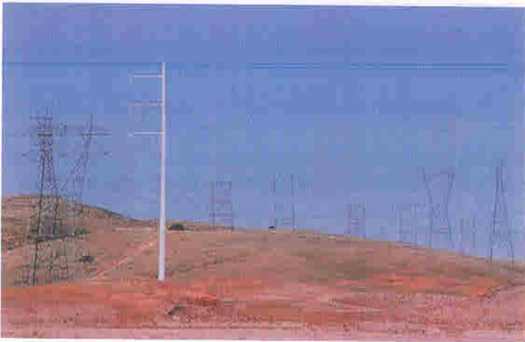
Figure B.3-2 View of the Antelope-Bailey Transmission Line Corridor Looking Southwest from the Proposed Substation Site.
