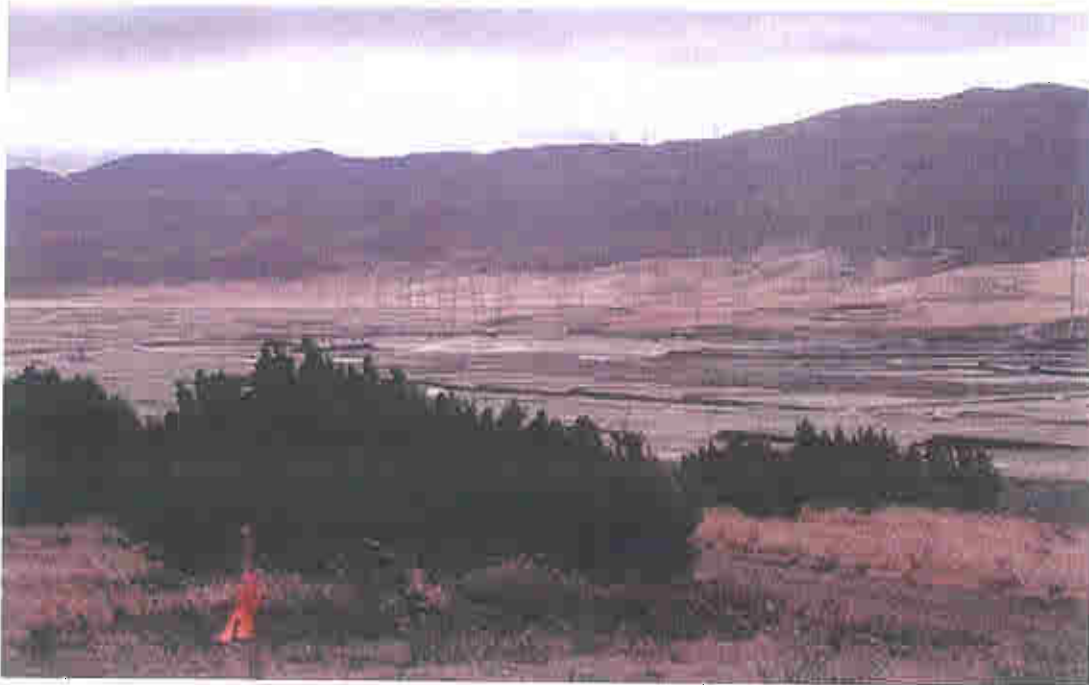
Figure B.3-1 View Looking Southeast Toward Development Area and the Antelope Bailey Transmission Line Corridor. Proposed Substation Site is Located in the Center of the Photograph.
