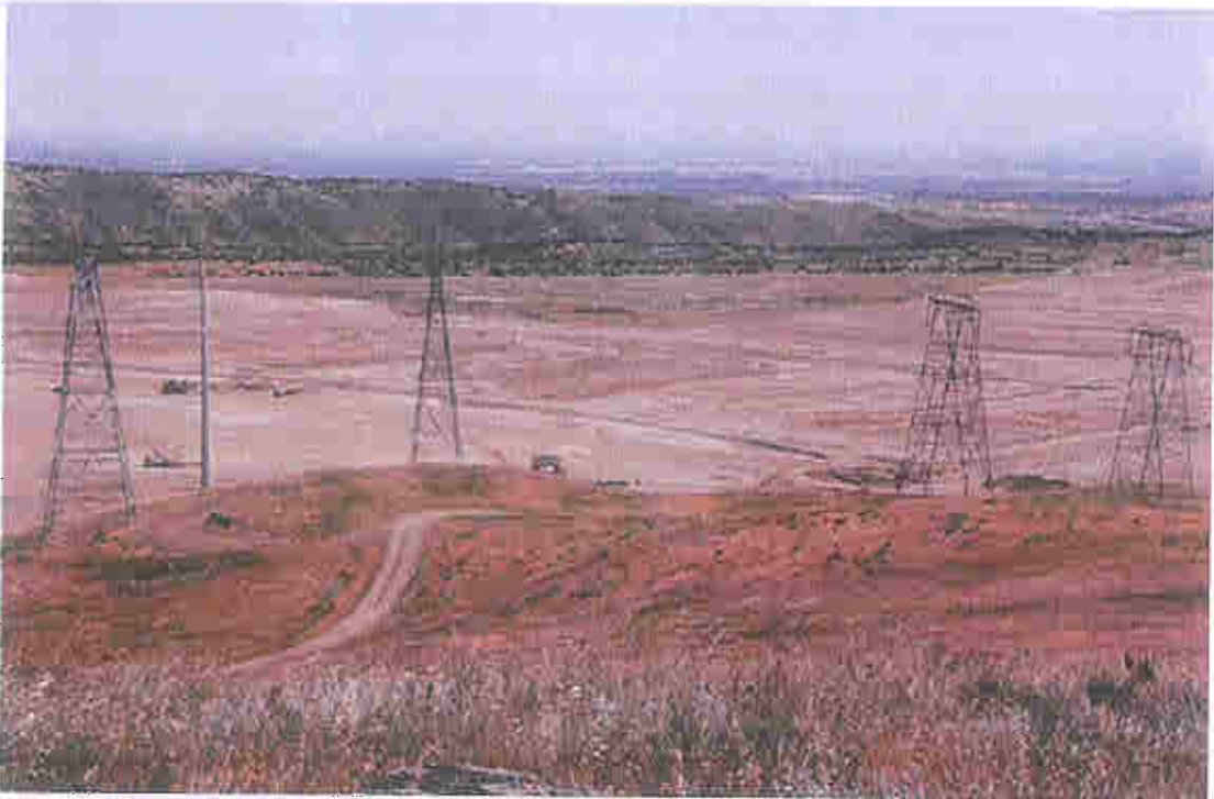
Figure B.3-3 View Looking Northeast Across the Antelope-Bailey Transmission Line Corridor and Ritter Ranch Development. Proposed Substation Site is located in the center of the photograph.
