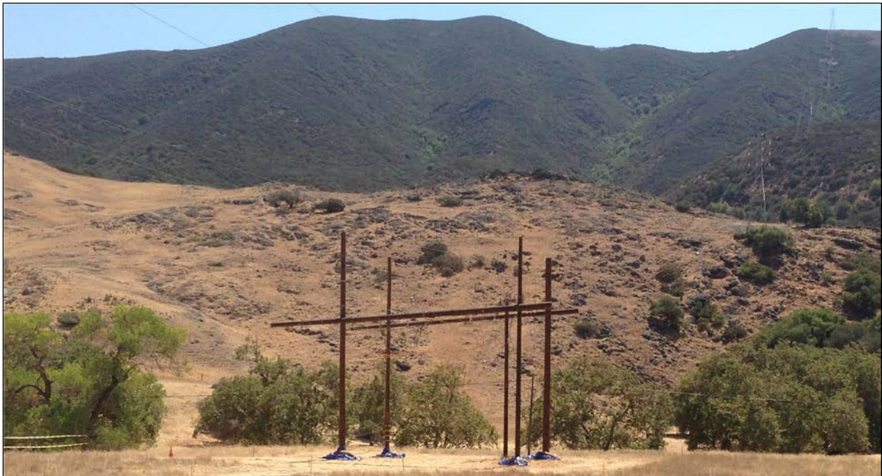
Figure 2.6-2 Horizontal Pole Guard Structure
