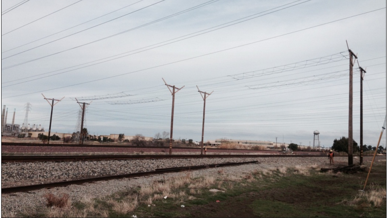
Figure 2.6-3 Type "Y" Guard Structure
