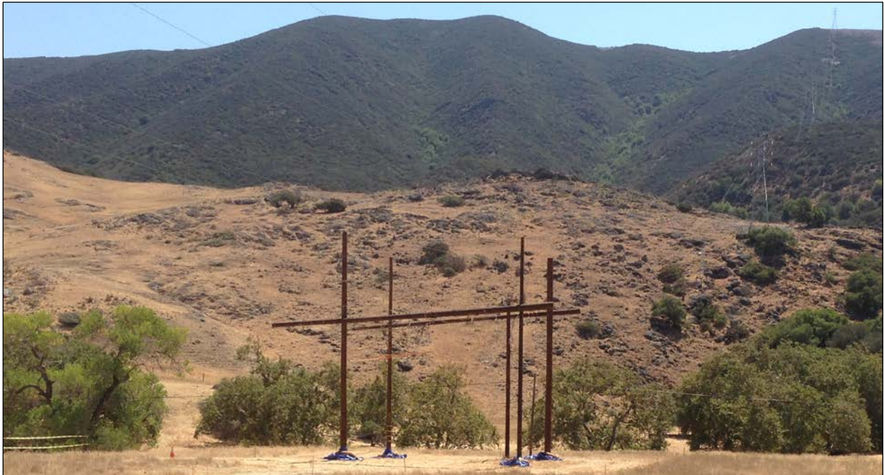
Figure 2.6-2 Horizontal Pole Guard Structure
