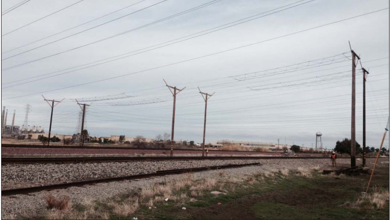
Figure 2.6-3 Type "Y" Guard Structure
