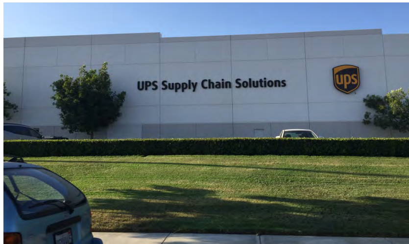
EXHIBIT C. VIEW OF ONE OF THE INDUSTRIAL BUILDINGS NORTH OF LANDON DRIVE
